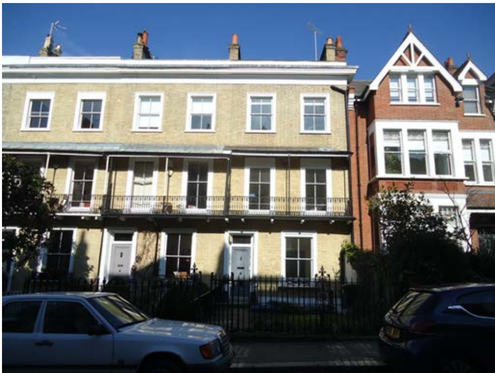
Figure 1: Street elevation of no. 40 Richmond Hill (right of centre, facing)
