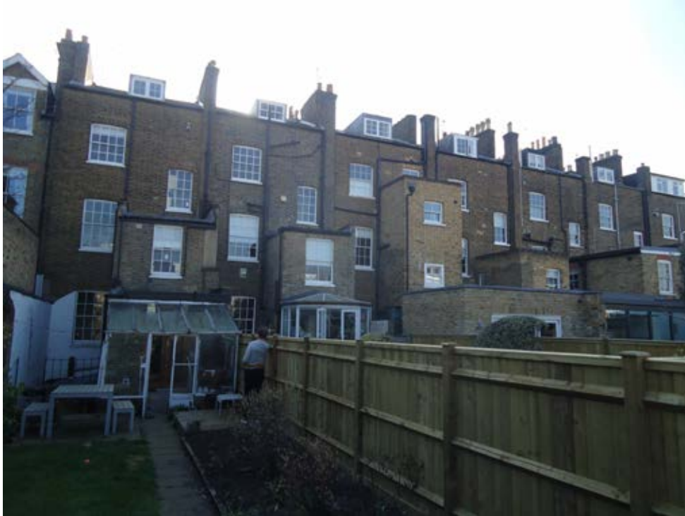
Figure 2: Rear of terrace nos. 28 to 40 Richmond Hill. No. 40, the Site, to the far left facing
