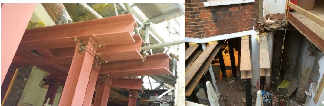
Figure 1 Example of needling to existing wall/bay window
