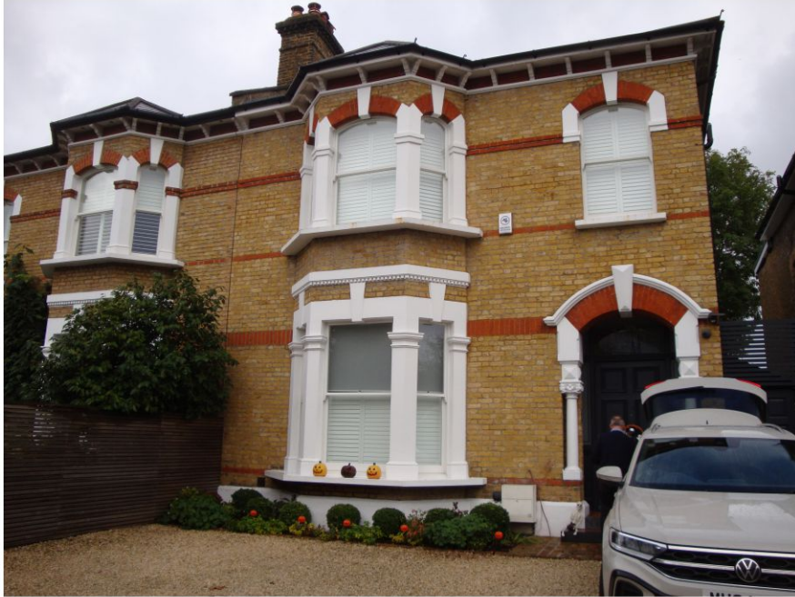
Front Elevation – general view
