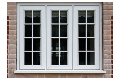
6. Windows / doors Timber with white finish. Seals and spacer bars in white
