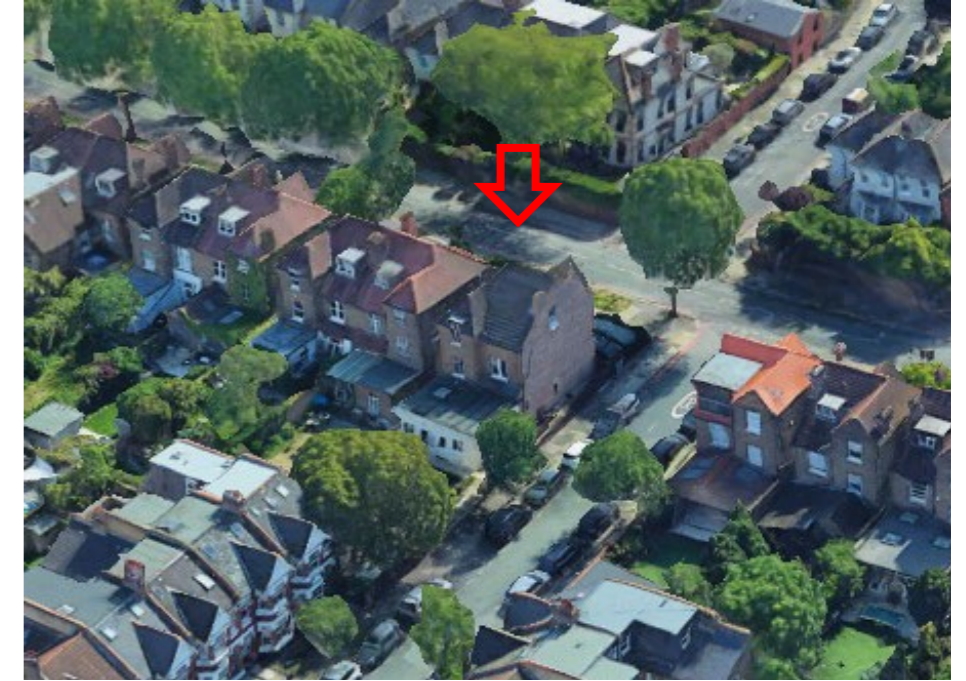
Fig 4 / This view of the rear of the property shows how the rear elevation isn't especially light or open feeling. We believe our design works with these constraints and adds the modest extension to connect to the garden.
