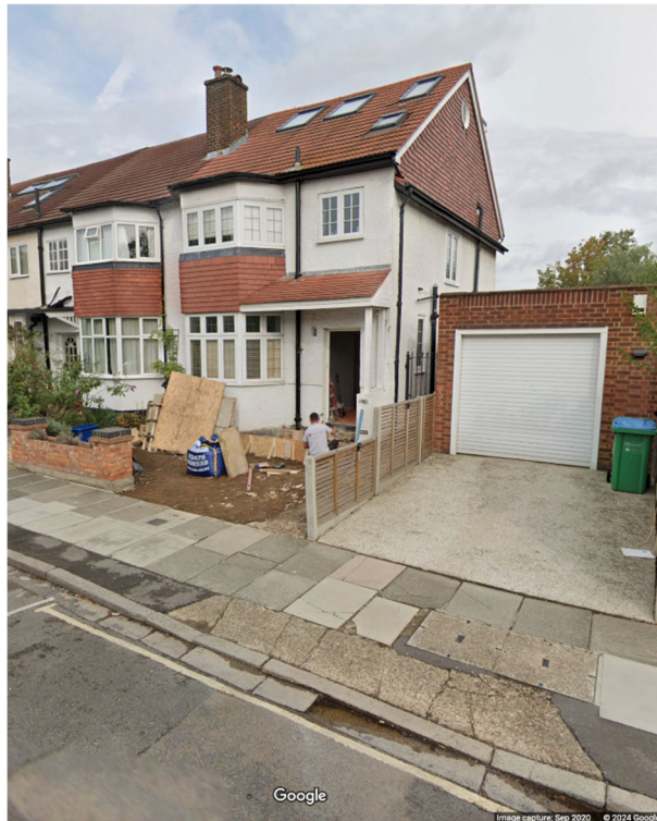
Figure 2; Front view of No. 44 showing the current canopy.
