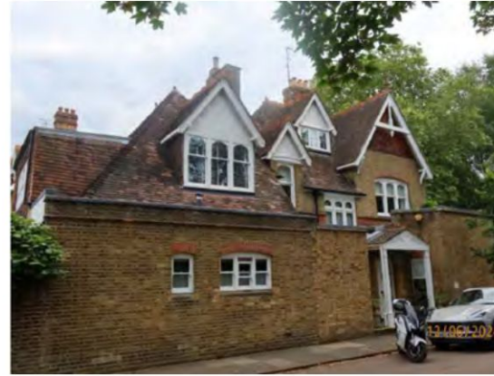
c) Flank façade of Thornfield from Woodlands Road.
