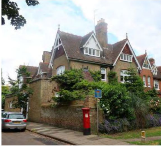
a) Thornfield front and flank façades.
