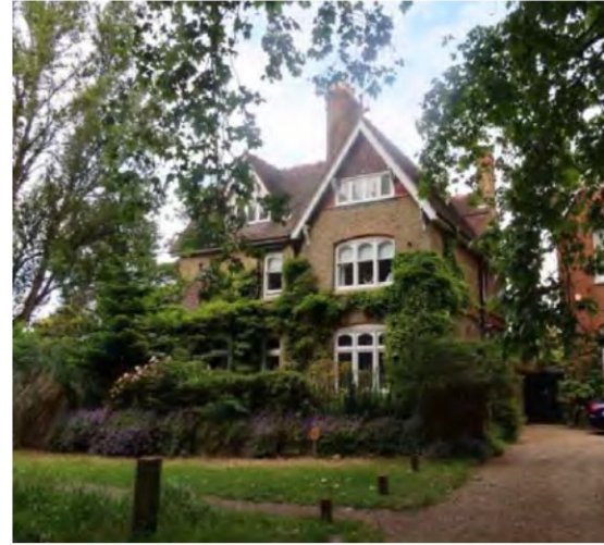
b) Front façade of Thornfield from Vine Road.
