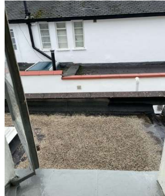
Item 6, = Inside access. Outside = Onto felt flat roof to protect, guarding rails required.
