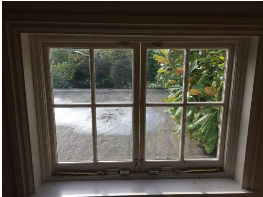
Figure 100: Side window to Bedroom 1
