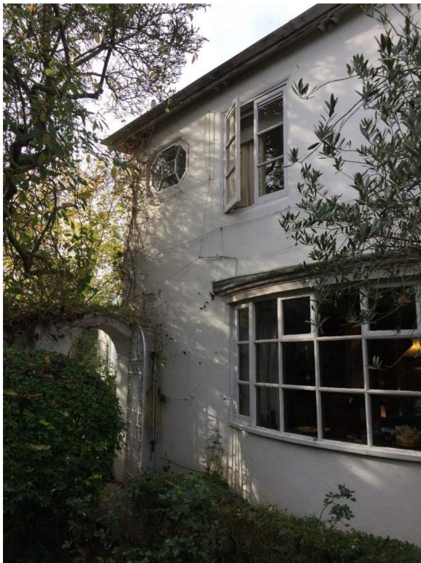
Figure 55: Rear elevation with 20 th century bow to Kitchen
