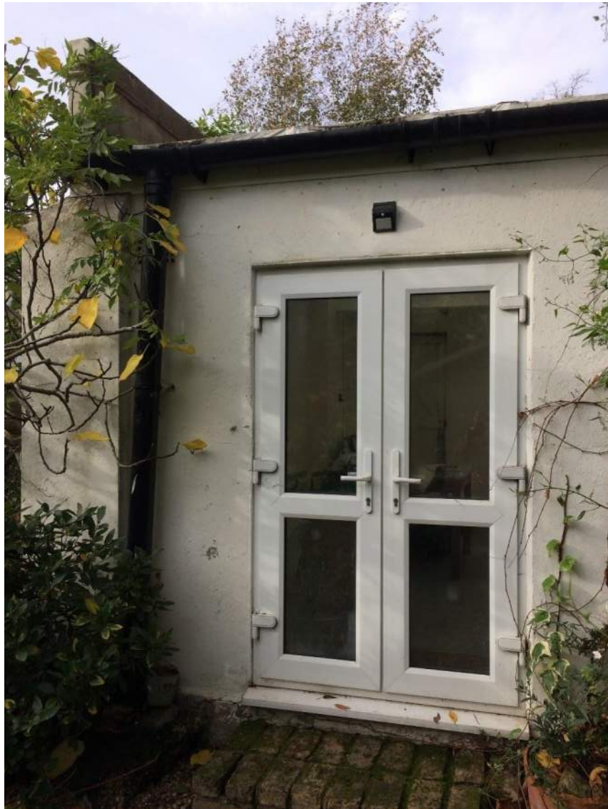
Figure 123: Double doors to rear of Garage
