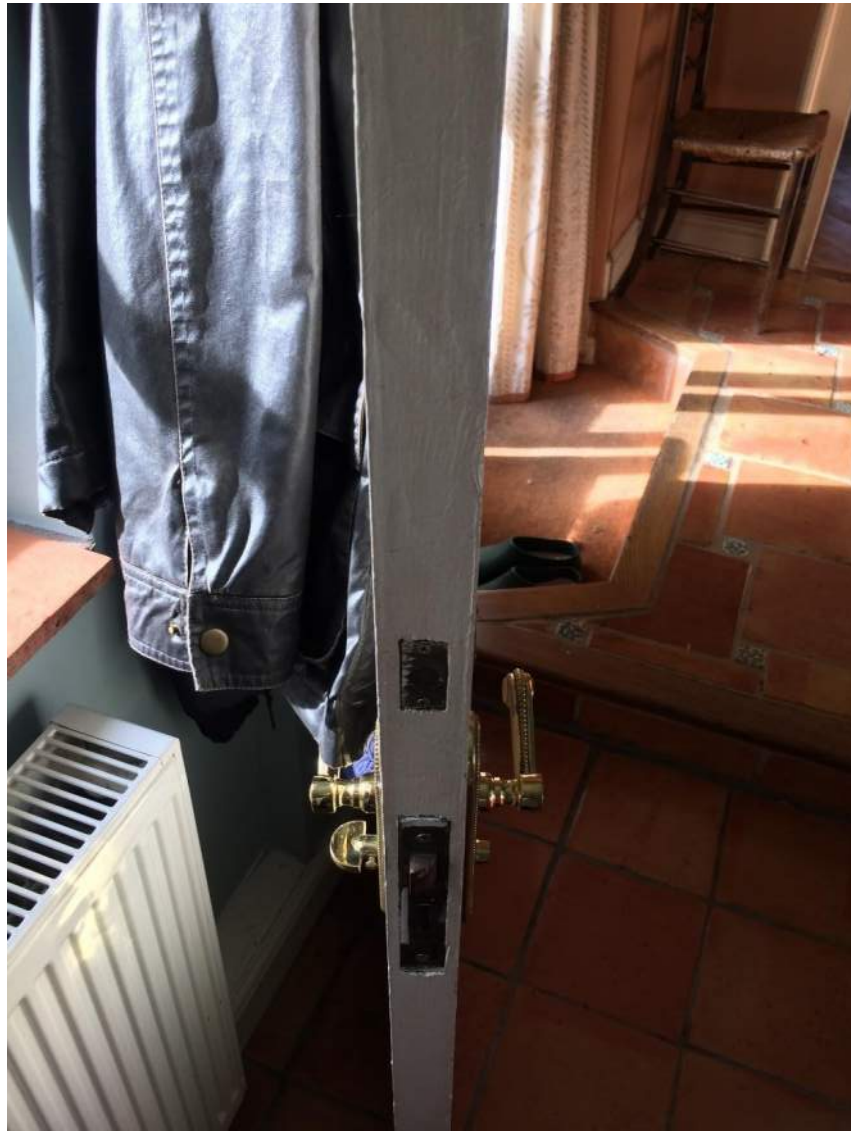
Figure 92: Modern door to W.C.
