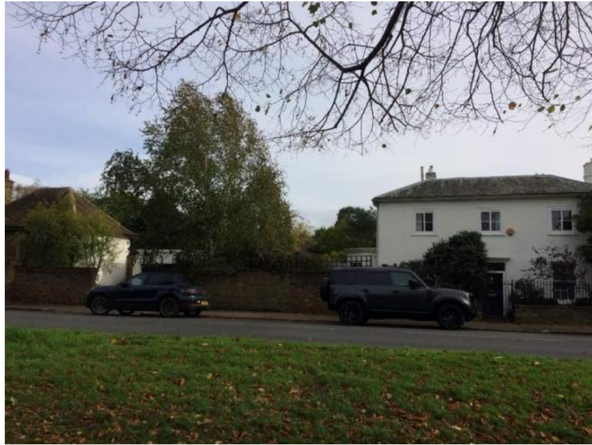
Figure 127: Fox House and Camilla Cottage, left
