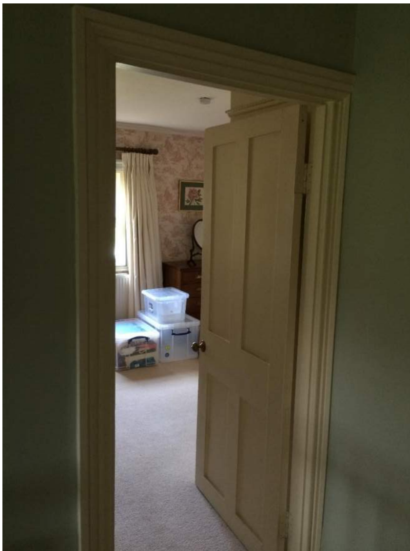
Figure 112: Door and partly cut or obscured architrave to Master Bedroom
