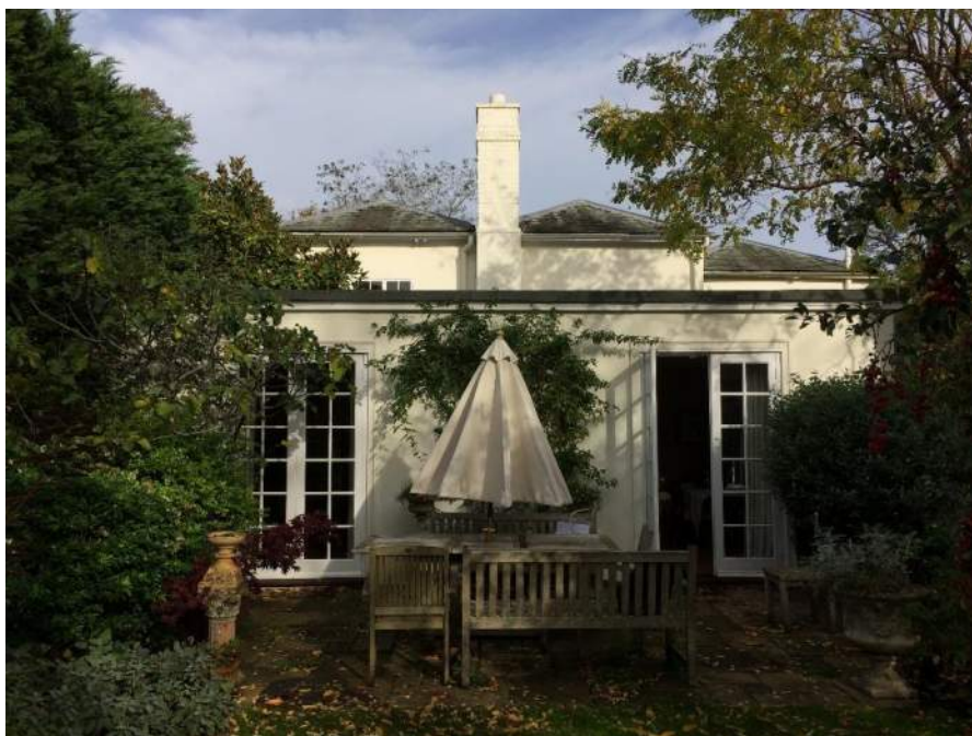
Figure 50: Mid-20 th century extension
