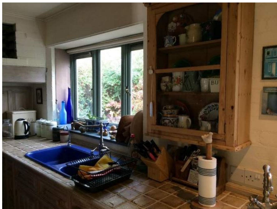
Figure 86: Three-light casement in Kitchen
