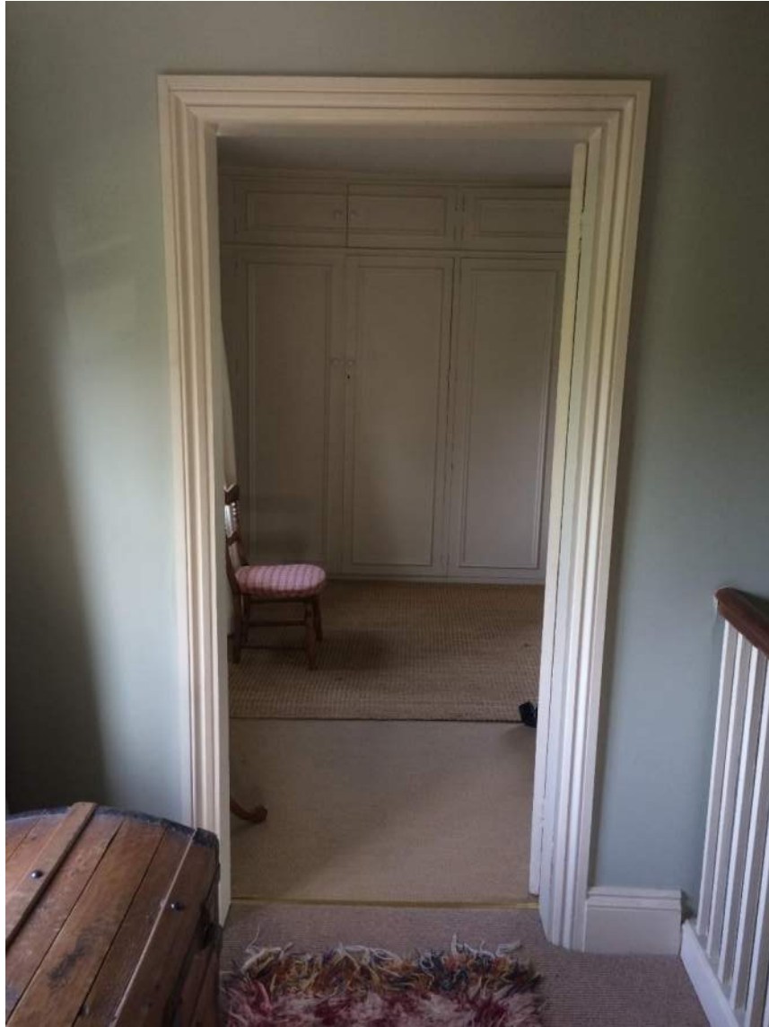
Figure 102: Landing and modern cupboards to Bedroom 2
