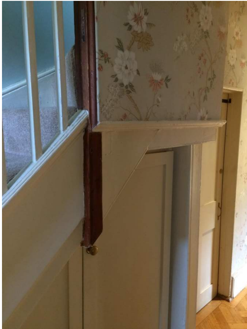
Figure 82: Reeded closed stringer to staircase with modern newel drop
