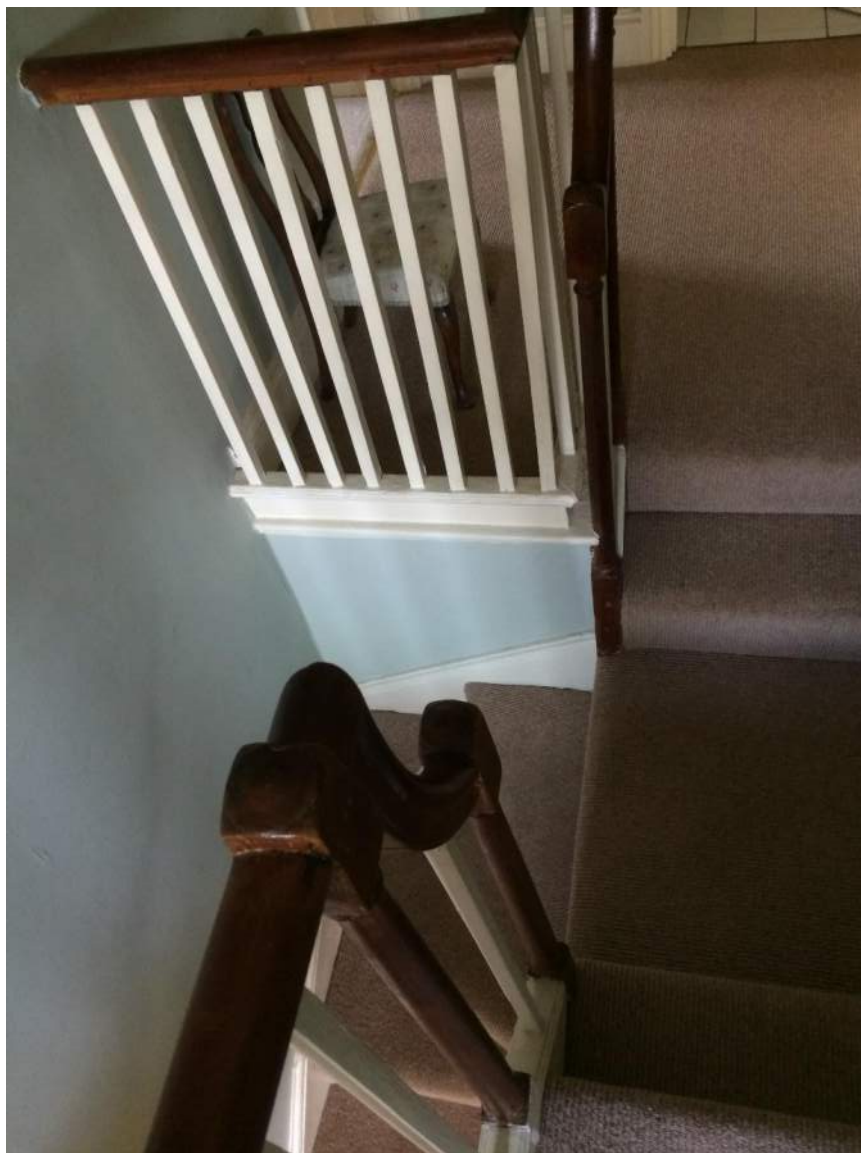
Figure 107: Handrails and newel posts to first floor
