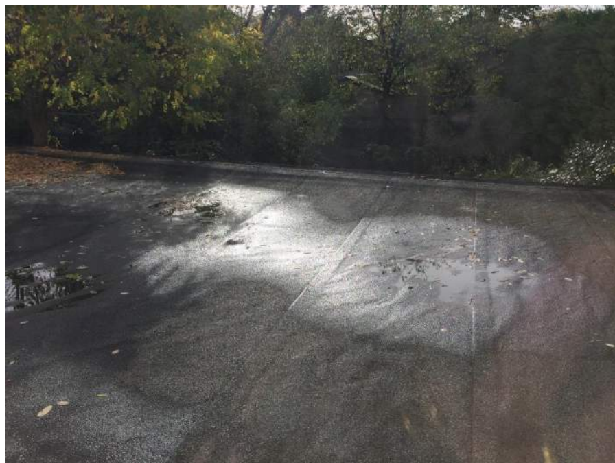
Figure 101: Felt flat roof to mid-20 th century Drawing Room extension
