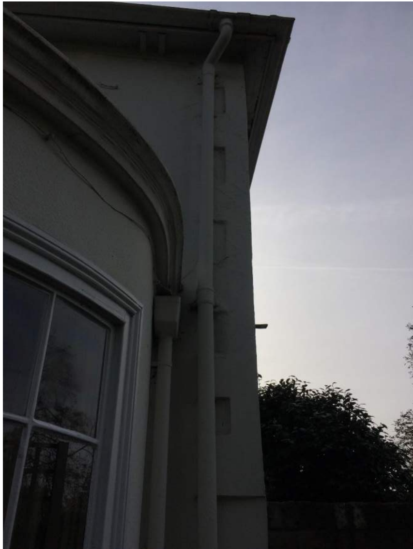
Figure 61: Quoins effect in stucco to corner of north-east elevation
