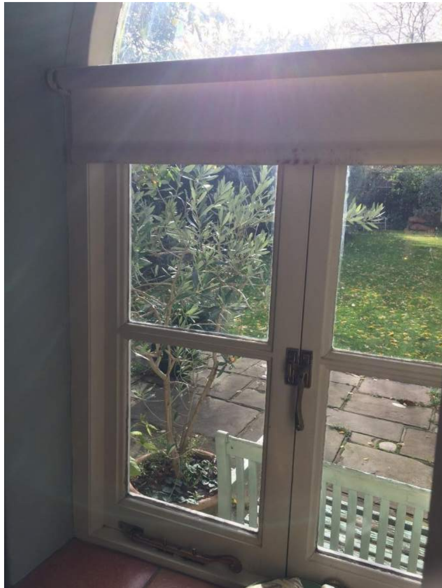
Figure 93: Modern casement to W.C.
