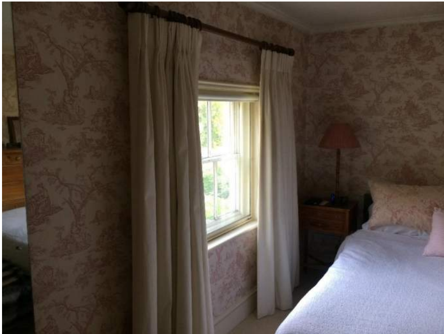
Figure 115: Sash window to north-east elevation
