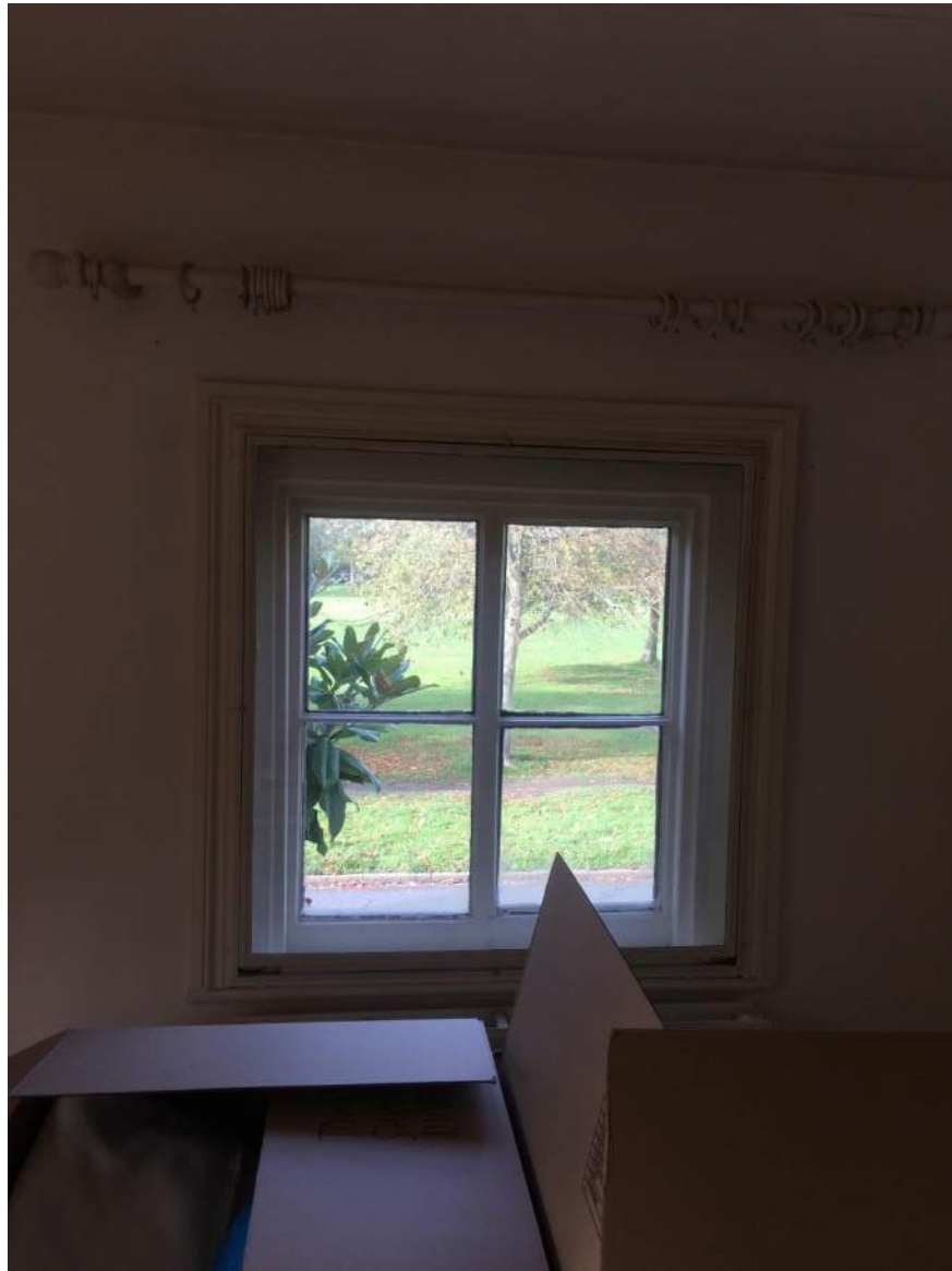
Figure 99: Casement (sealed) to Bedroom 3
