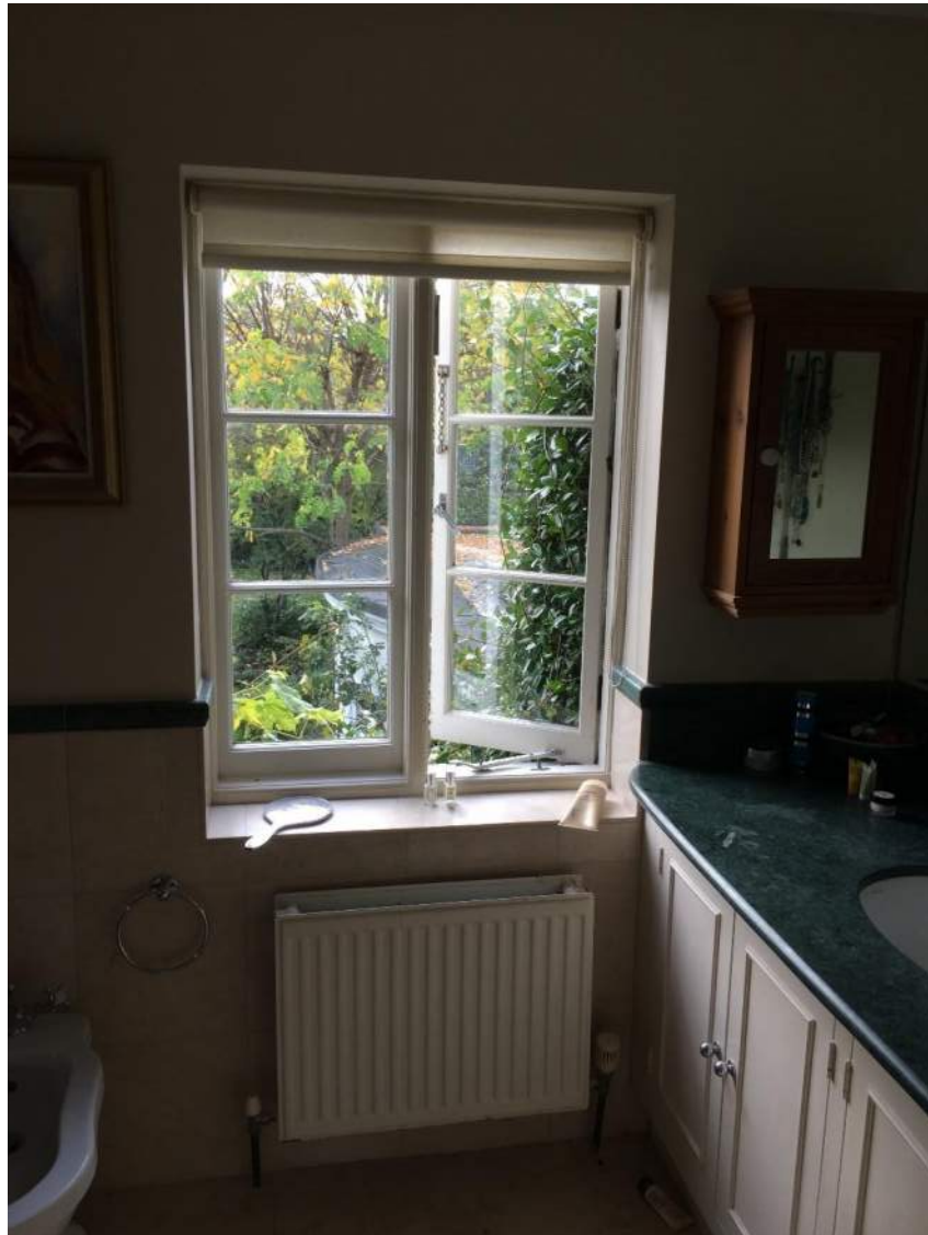
Figure 120: Modern casement to Principal Bedroom Ensuite
