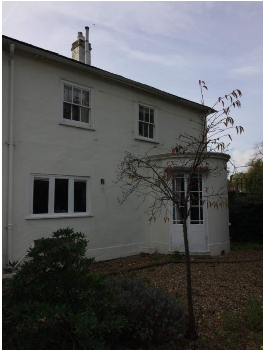
Figure 60: North-east elevation with bow added in the mid-20 th century
