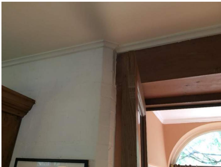
Figure 89: Brick chamfer edge detail to W.C
