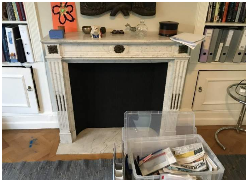
Figure 73: Existing fireplace and hearth (modern) to Study
