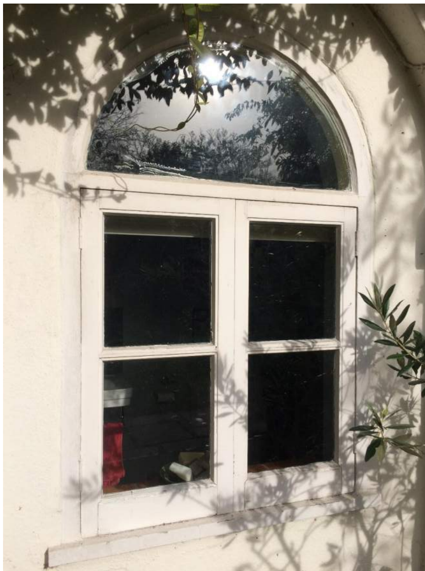
Figure 54: Modern casement to W.C.
