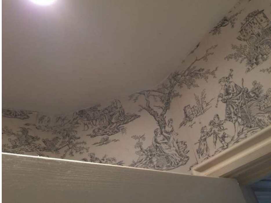
Figure 111: Realigned wall to main Bathroom
