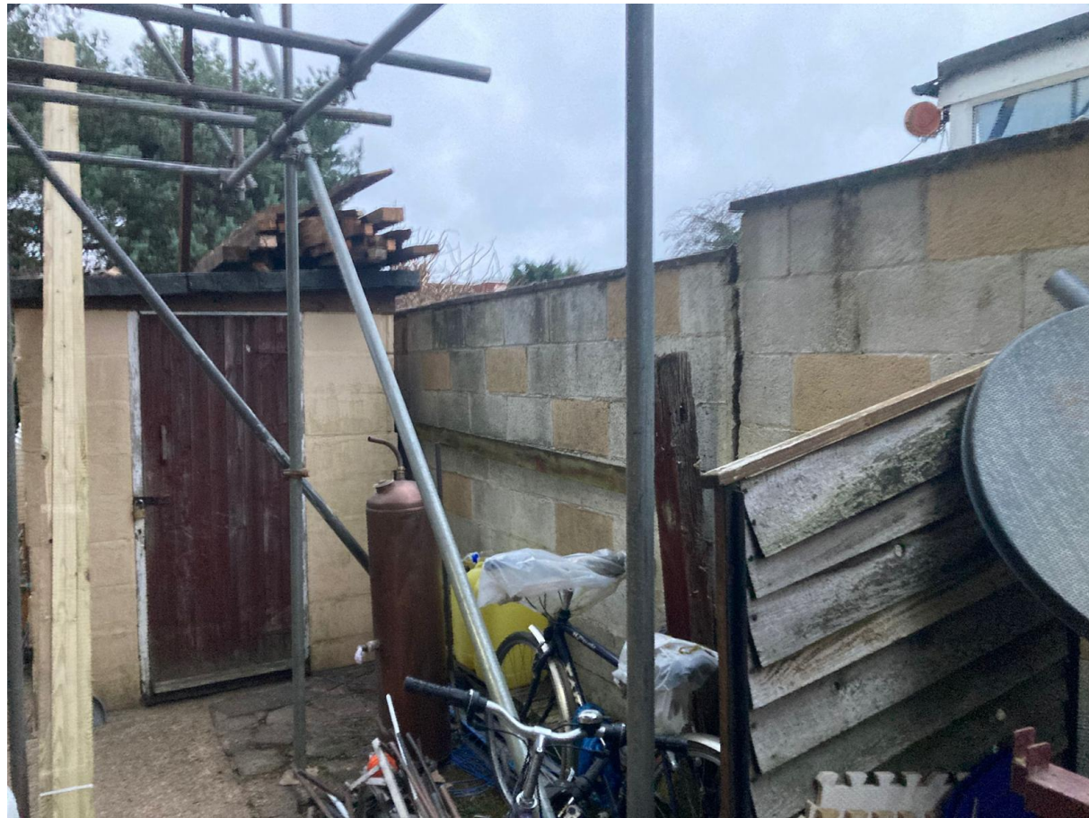
View of the existing outbuilding
