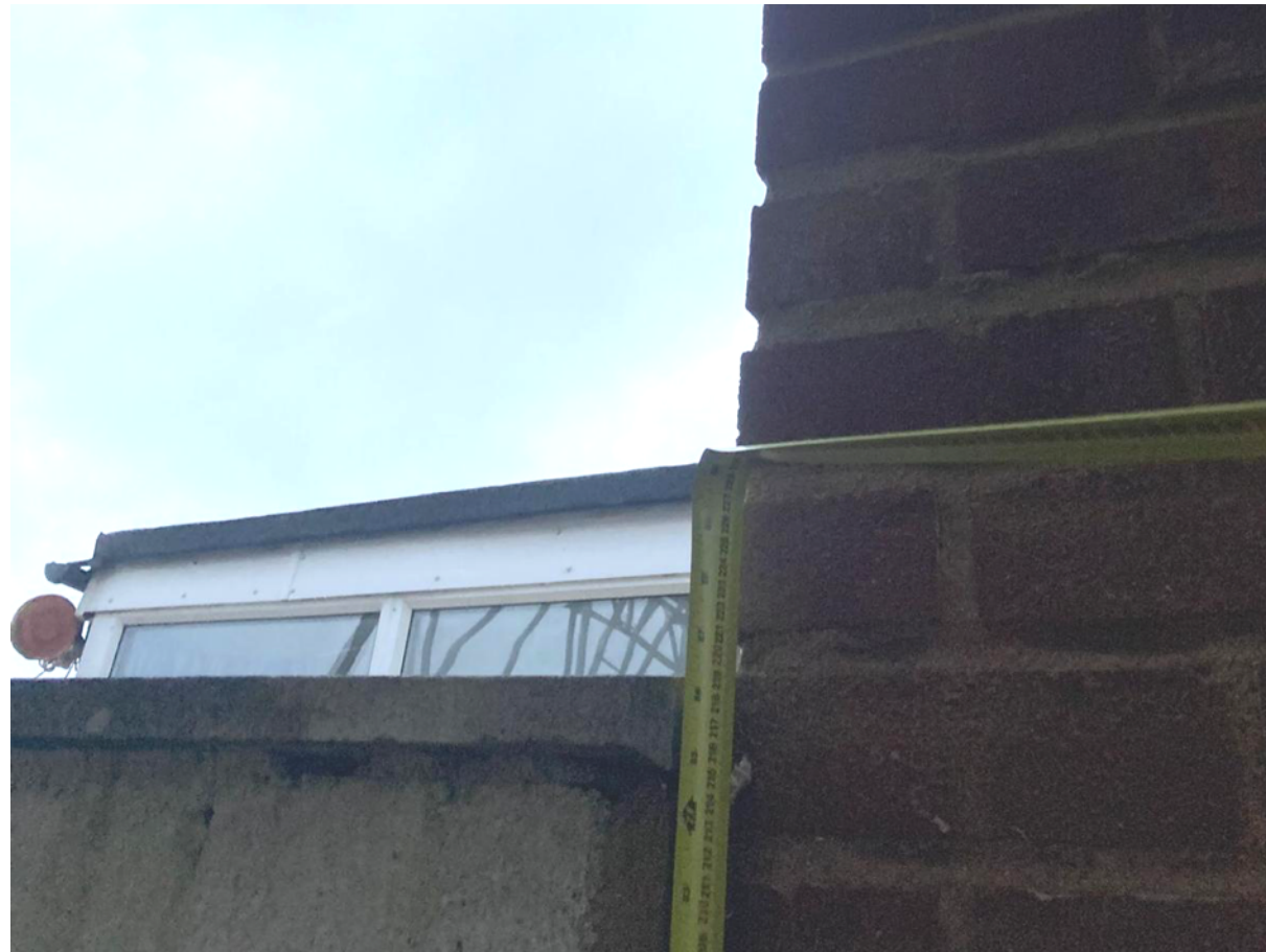
View of the existing outbuilding
