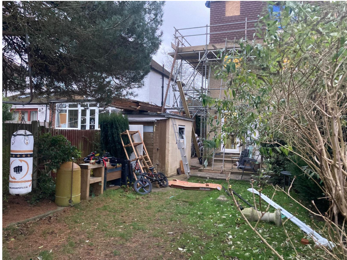
View of the existing outbuilding
