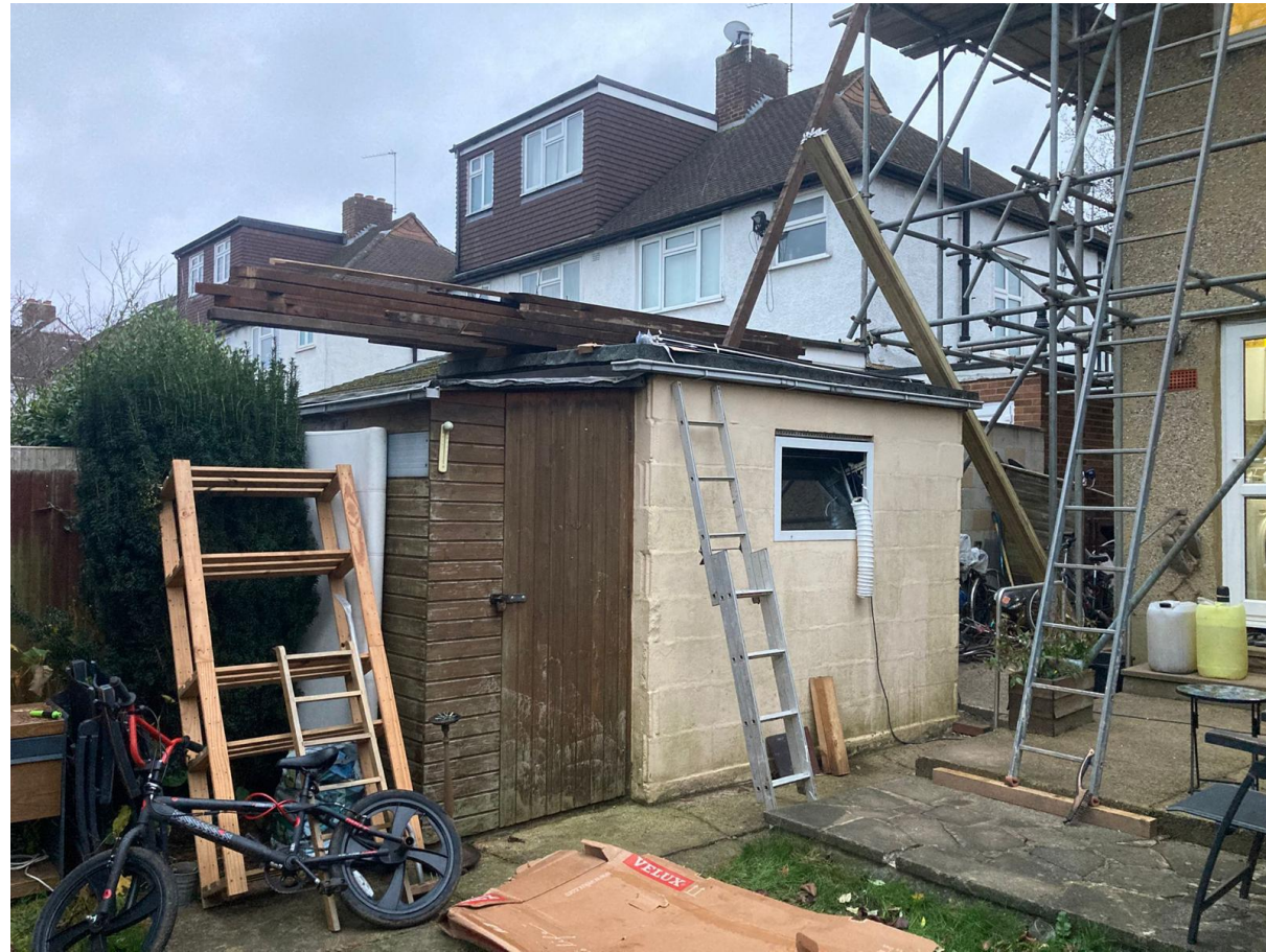
View of the existing outbuilding
