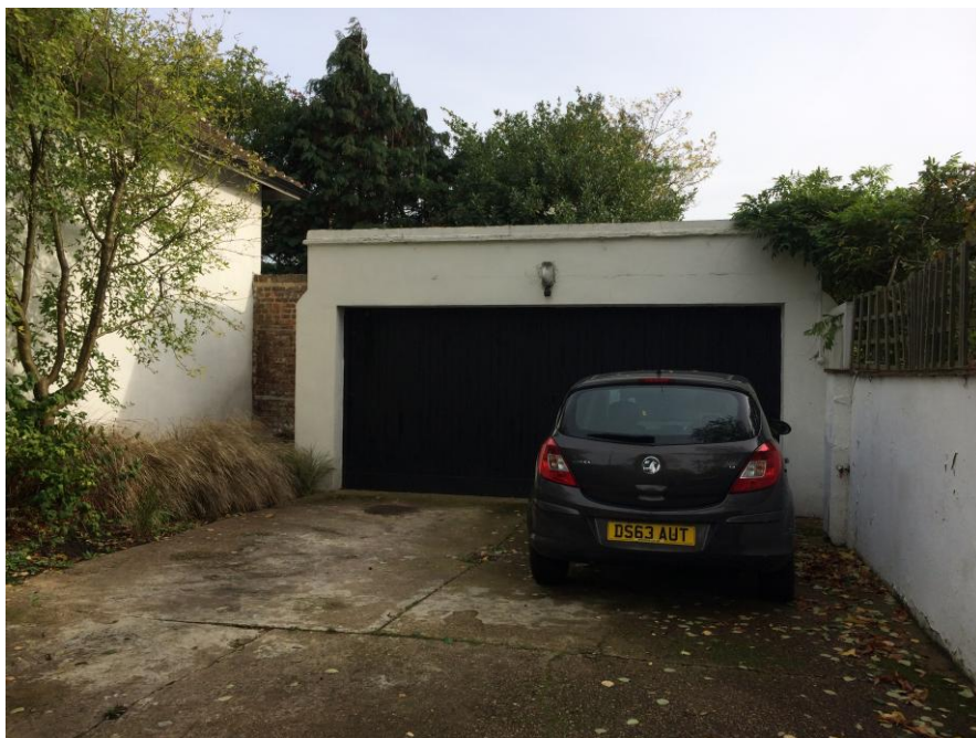
Fig. 04 Parking area with concrete hardstanding
