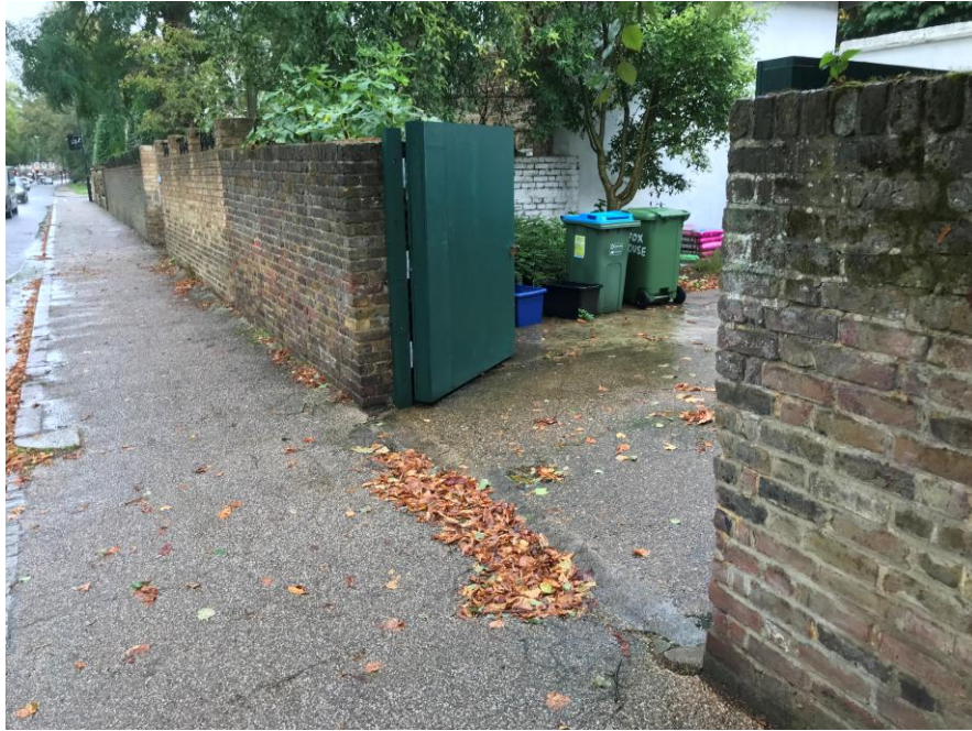
Fig. 03 Existing opening with timber gates
