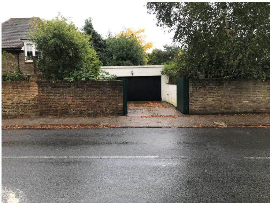
Fig. 02 Existing opening with garage beyond
