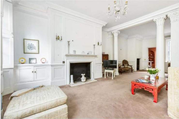
5 Old Palace Terrace – Existing enlarged opening between front and rear room with Corinthian columns.
