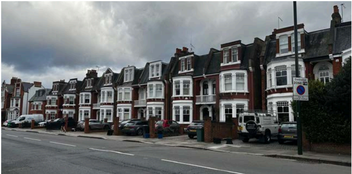
View of the row of semi-detached houses at Wellington Road
