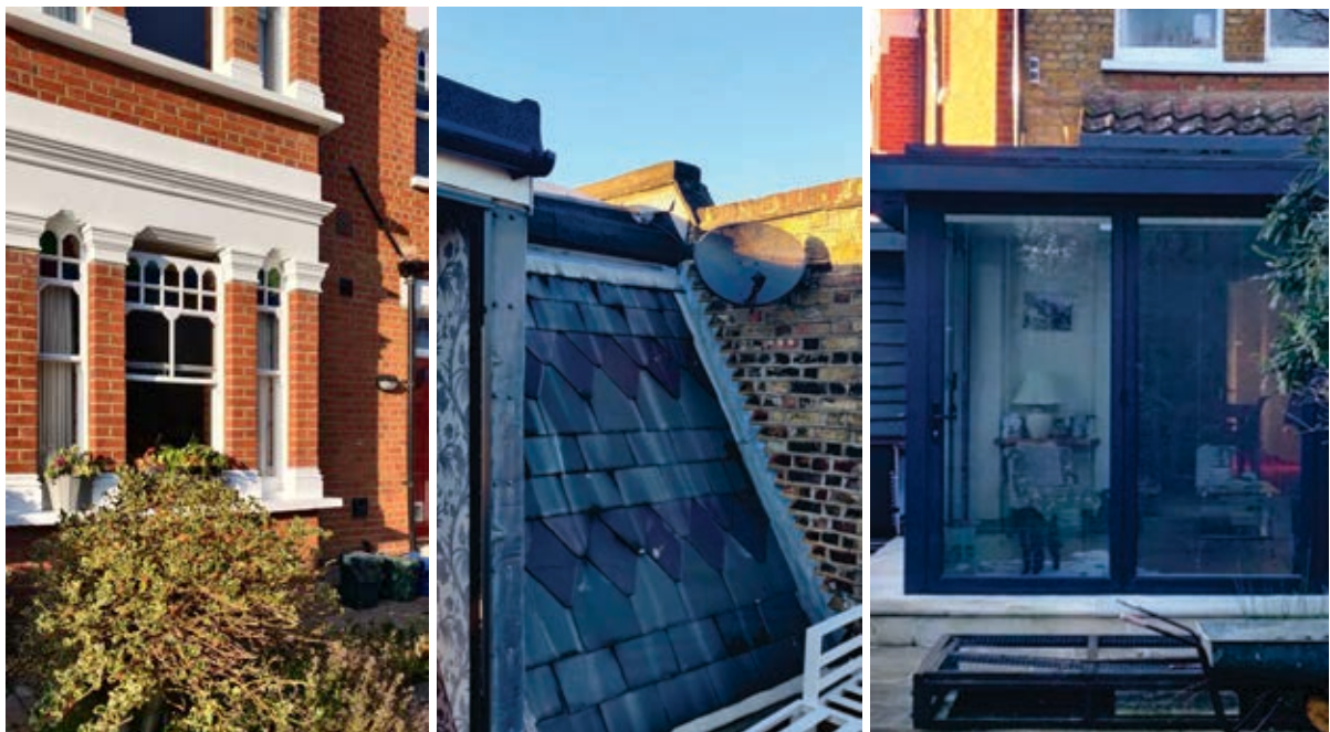
Material used at the existing dwellinghouse
