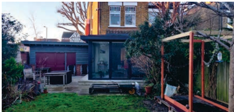
Rear view of the existing extensions.
