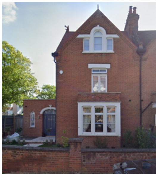
Approved extension to 20 Waldegrave Gardens, as constructed
