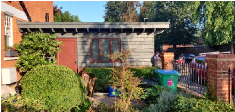
Front view of the existing side extension.
