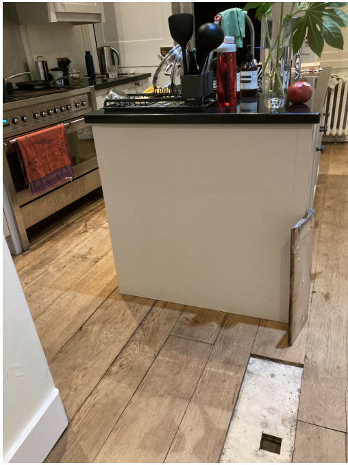
1 - Photo - Showing engineered flooring sample location in Kitchen
