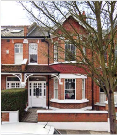
Front / north elevation, facing Palmerston Road
