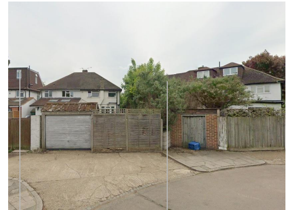
f.Rear of no. 36 + 38 Rivermead's Avenue
