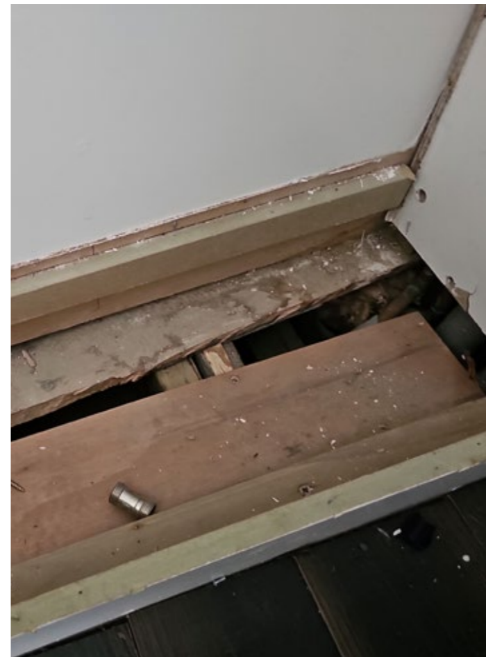
Modern plasterboard finishes in store.
