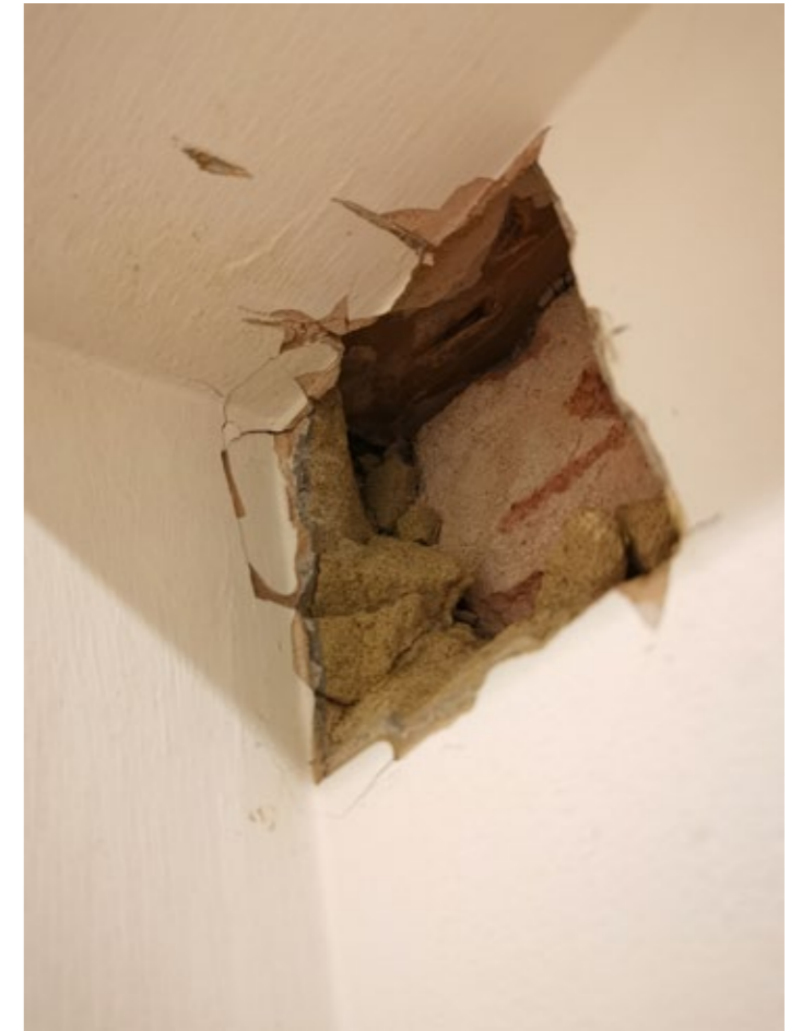
Opening up works to both sides of the recess (shown in the image to the left) have revealed the presence of modern plaster and block work likely installed in the 1960s to block up the original opening seen by the original timber lintel, also visible.
