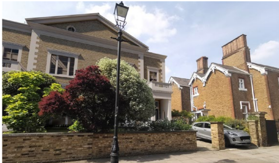
Existing side view of No.10 from Pembroke Villas
