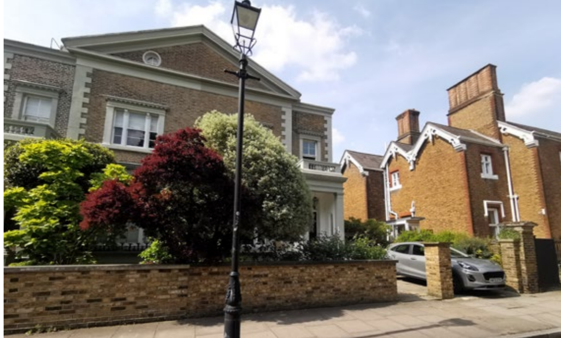
10 Pembroke Villas front view
