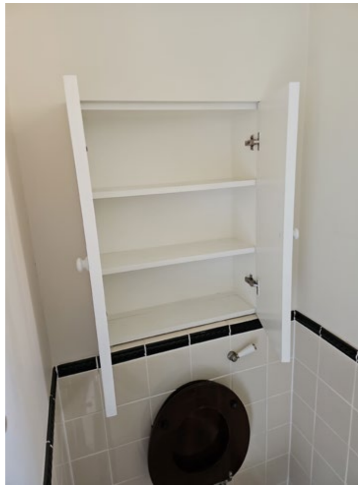
Modern joinery and plasterboard in WC
