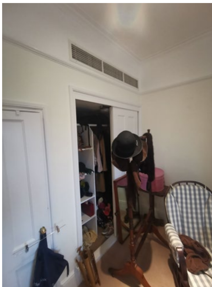
Modern partition accommodating built-in wardrobe and air conditioning unit
