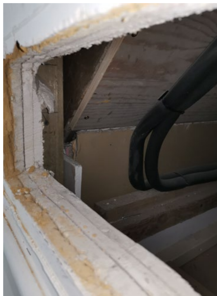
Modern plasterboard finishes around air conditioning grille
