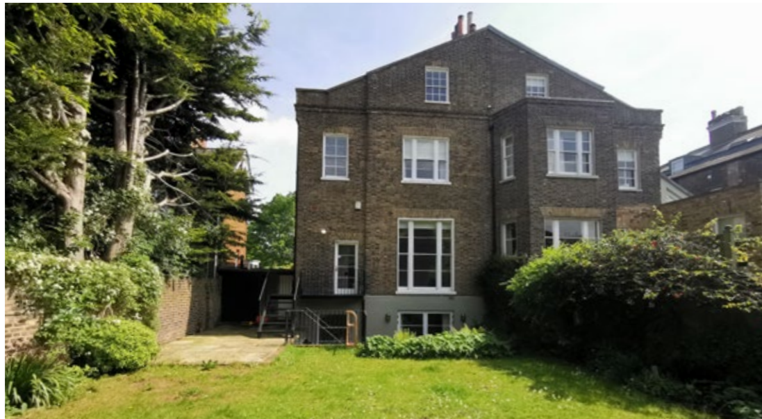
10 Pembroke Villas rear view
