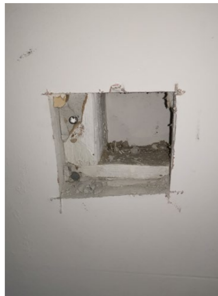
Modern plasterboard finishes in built-in wardrobe
