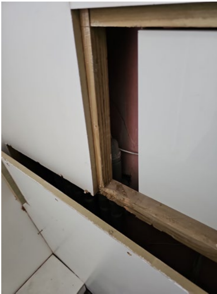
Modern fabric in existing store in hall, from 2011 works.
