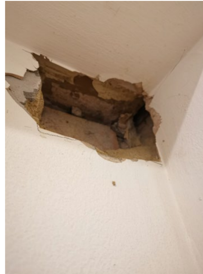
Opening up works to both sides of the recess (shown in the image to the left) have revealed the presence of modern plaster and block work likely installed in the 1960s to block up the original opening seen by the original timber lintel, also visible.
