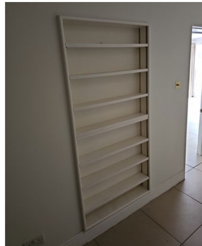
Original door opening to be reinstated.
