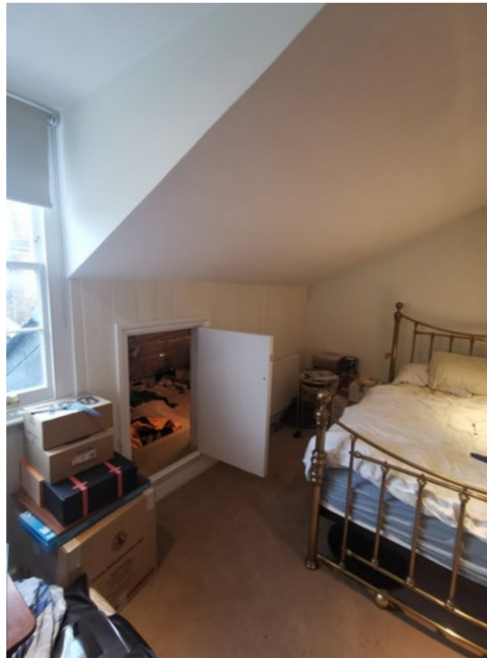
Wall panelling in bedrooms
