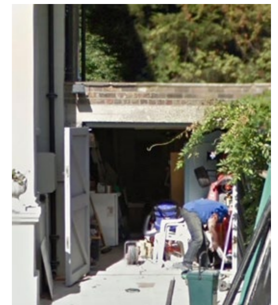
Image from 2012 showing the concrete lintel above No.10 garage doors
