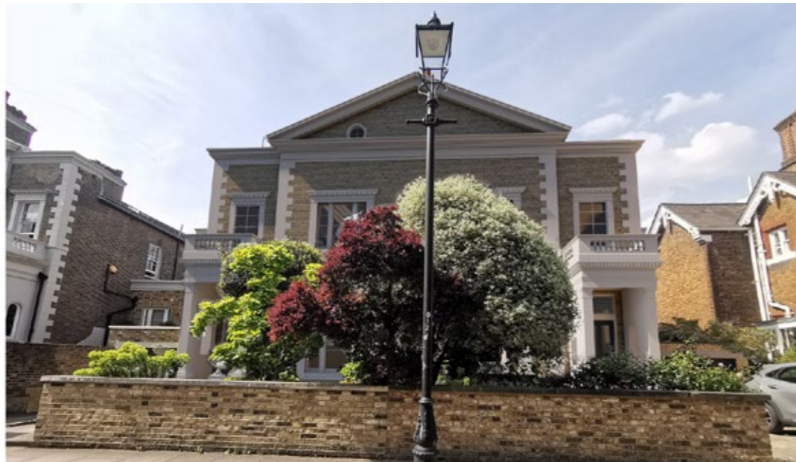
Existing front view of No.10 from Pembroke Villas
