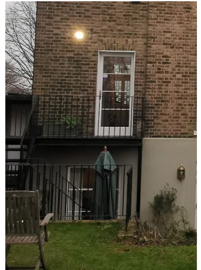
EXISTING VIEW FROM REAR GARDEN
