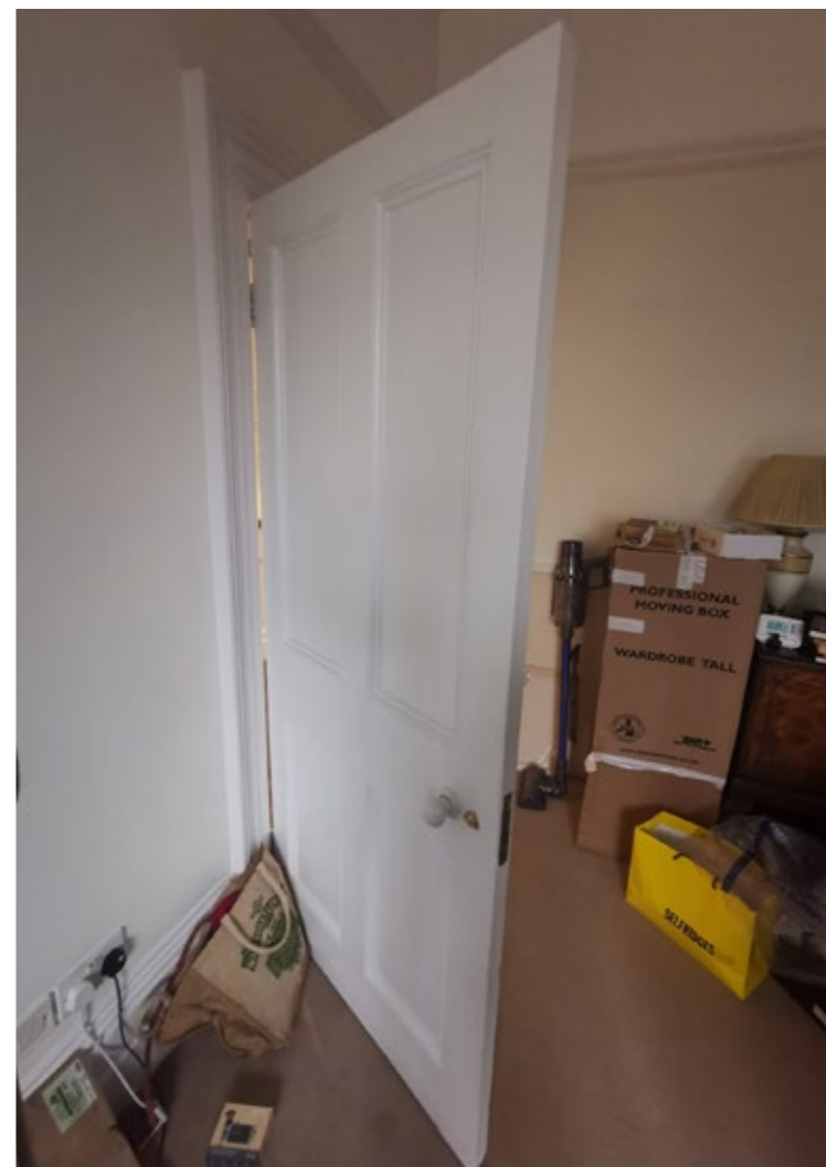
SIDE PROFILE OF ADJACENT DOOR D-022-03
