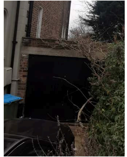
External view of garage door D-022-11
