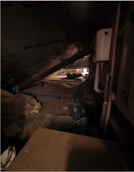
Existing eaves storage to bedroom 04
