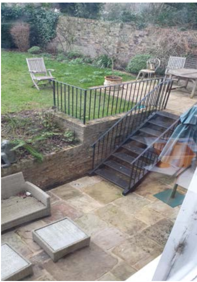
Existing patio, and level differences
