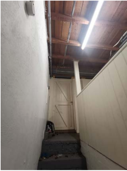
Existing entrance from garage
