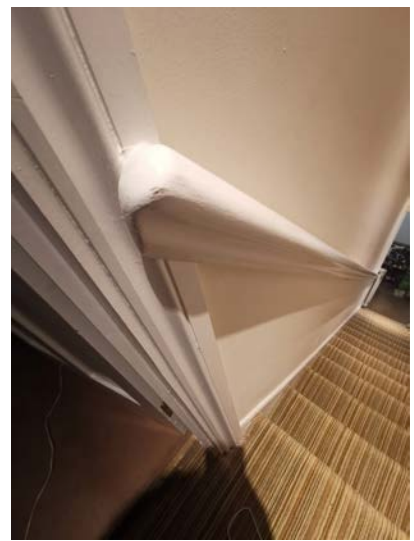
Existing balustrade and architrave details
