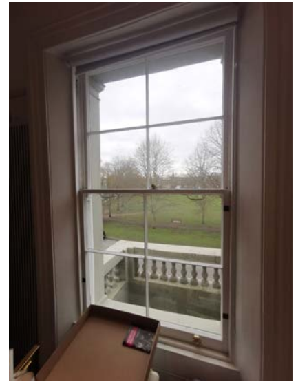
Existing window W-023-05
