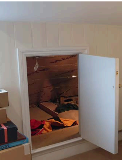
Door to eaves storage D-024-04
