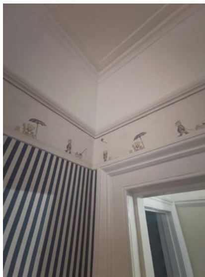
Existing cornicing and architrave details
