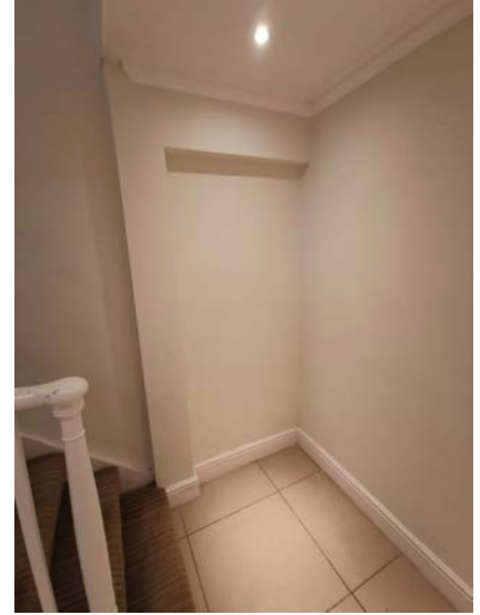
Existing partition where D-021-13 is to be reinstated.
