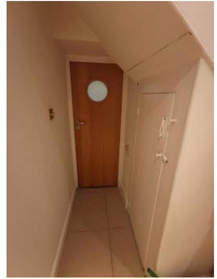
Existing modern D-021-01 entrance from garage to hallway
