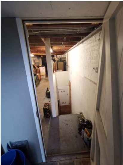
View from D-022-07 into the garage
