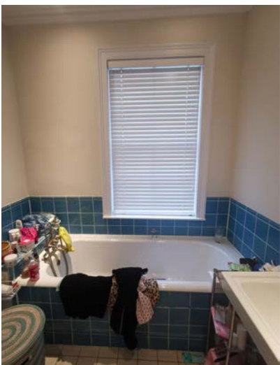
Existing window W-023-03
