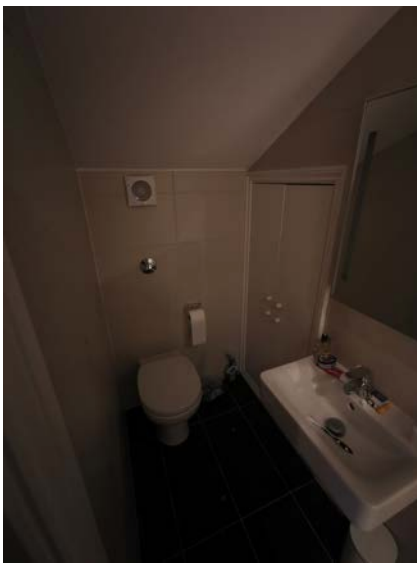
Existing shower room 02
