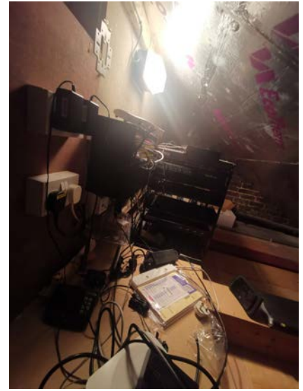
Existing eaves storage to bedroom 04
