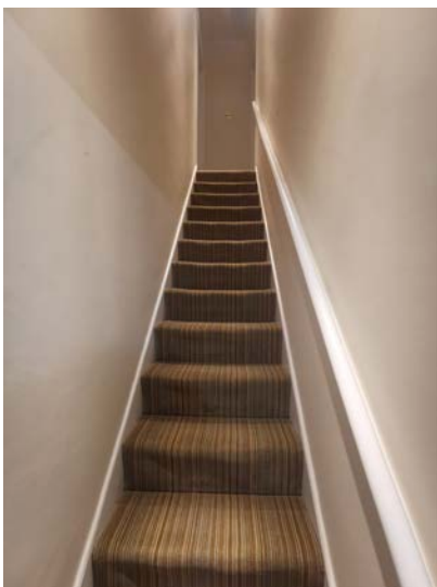
Existing staircase to second floor
