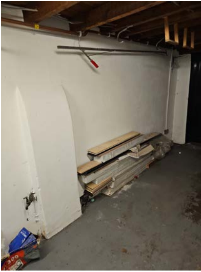
Inside the existing garage
