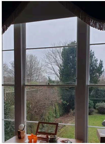
Existing window W-022-02
