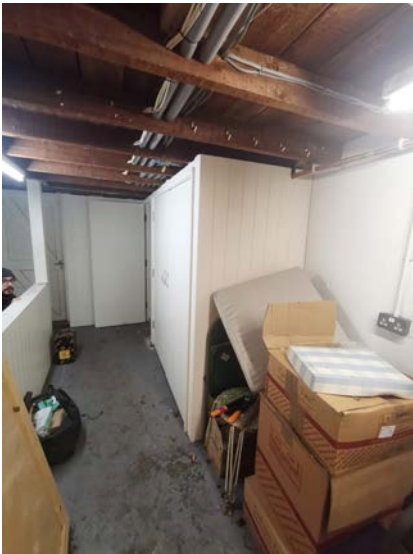
Existing entrance from garage
