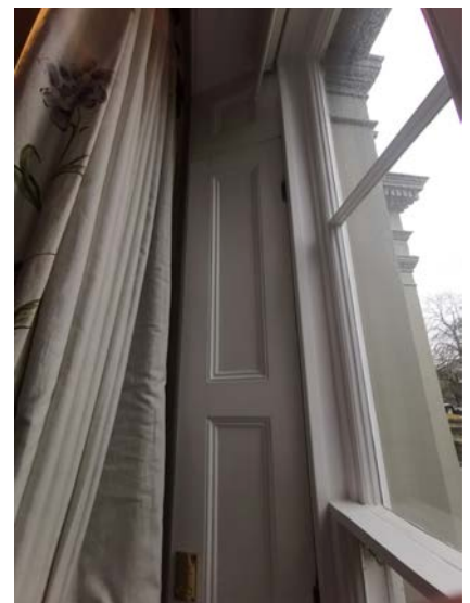
Existing shutter to W-022-01
