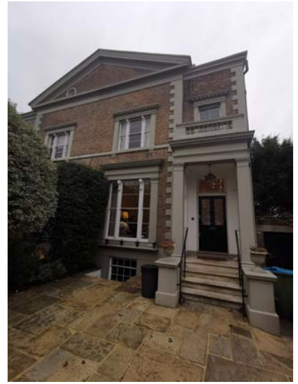
Existing paving to the front
