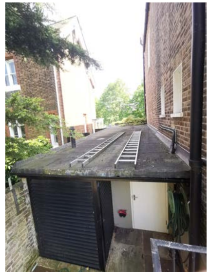
Existing roof finish of garage
