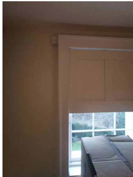
Existing window W-024-01
