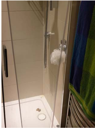
Existing shower room 01
