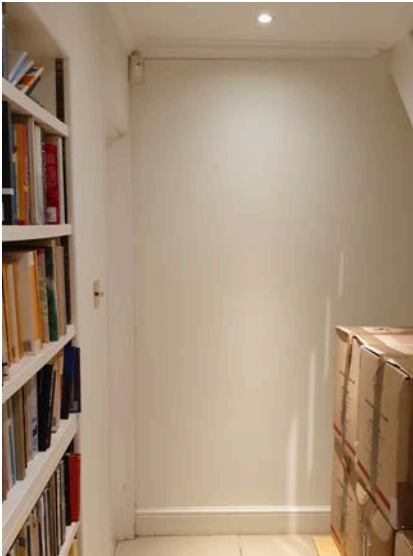
Existing partition between hallway and existing living room
