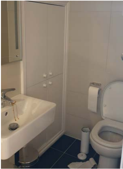
Existing shower room 01
