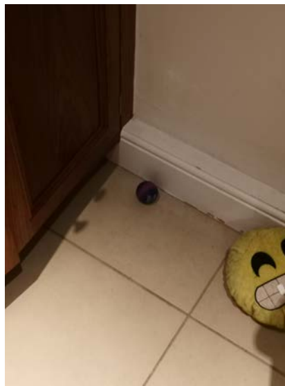
Existing skirting detail
