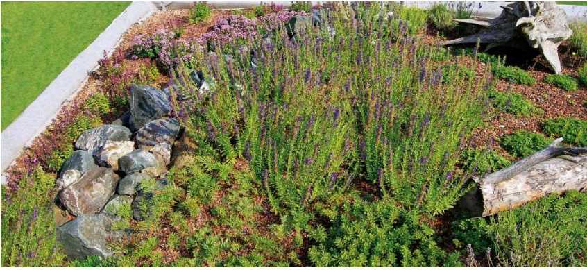
Image from www.zinco-greenroof.co.uk/systems/biodiversity-green-roof
