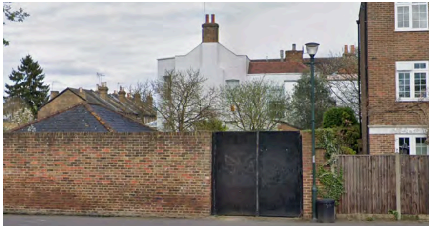
Fig.05 Gate Entrance, Back Lane
