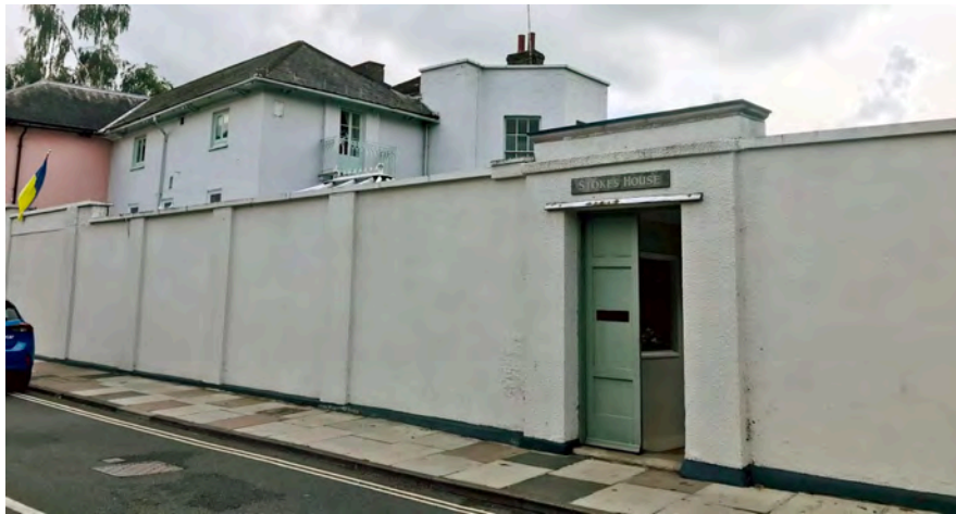
Fig. 04 Stokes House Entrance, Ham Street
