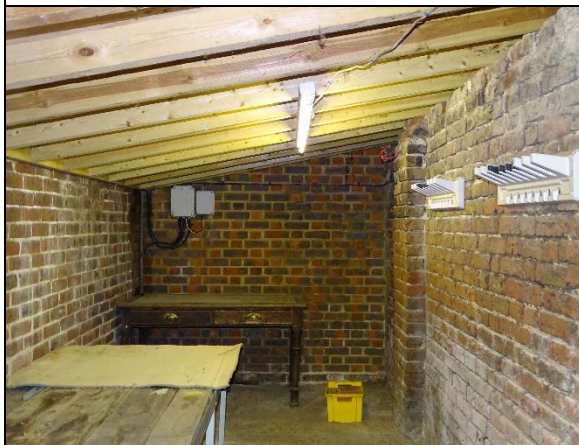
Photo 17: Internal view of outbuilding
