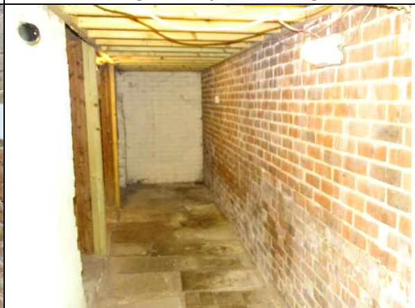
Photo 18: Internal view of outbuilding
