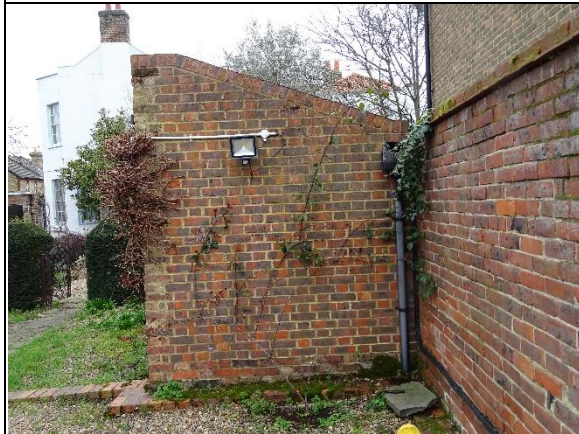
Photo 15: Northern face of storage building
