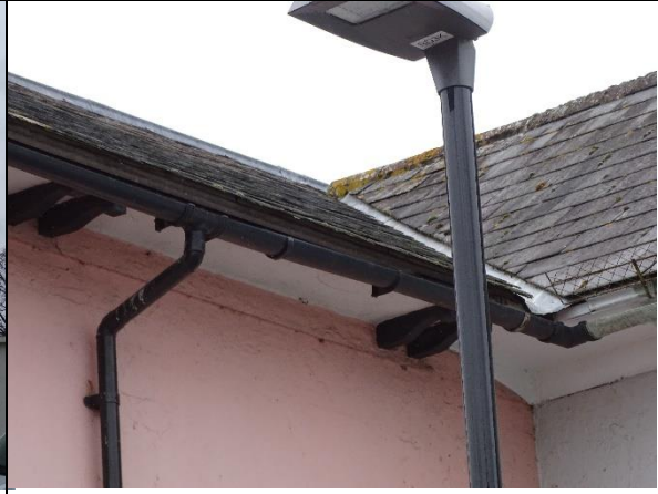
Photo 2: View of ridge and slate tiles at front of property
