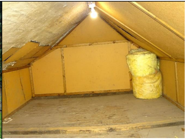
Photo 8: Interior of roof void, western end
