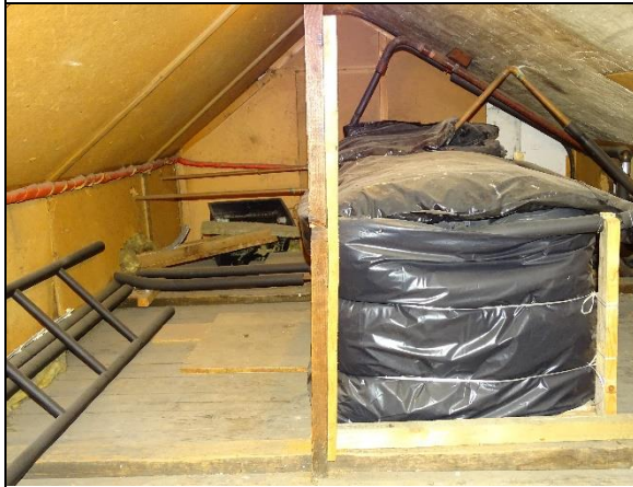
Photo 9: Interior of roof void, eastern end
