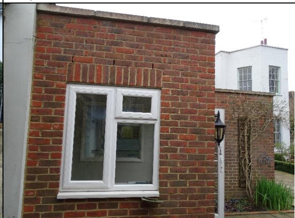
Photo 12: Eastern face of single storey building housing swimming pool
