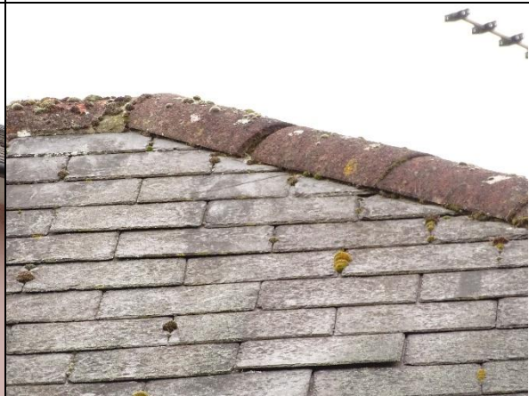
Photo 4: Brick ridge and slate tiles
