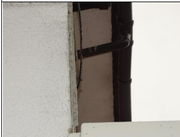
Photo 5: Soffits at front of main house
