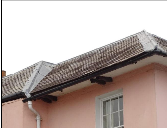
Photo 3: Recent well-sealed flashing on ridges, and intact soffits
