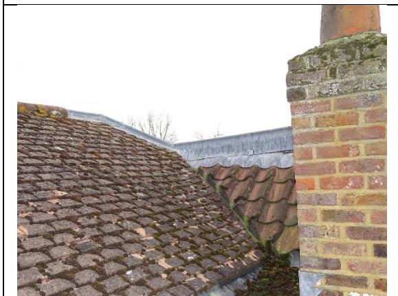
Photo 23: Brick chimney with evidence of recent re-pointing
