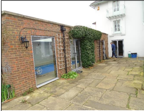
Photo 13: View of swimming pool building in relation to Stoke House
