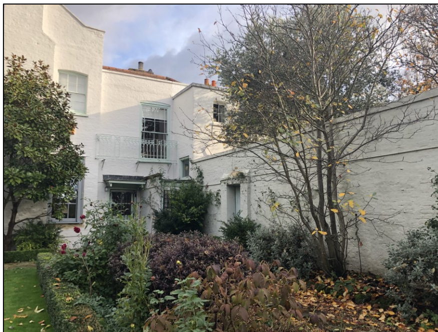
Plate 6: View of west-facing elevation showing door to the entrance hall.
