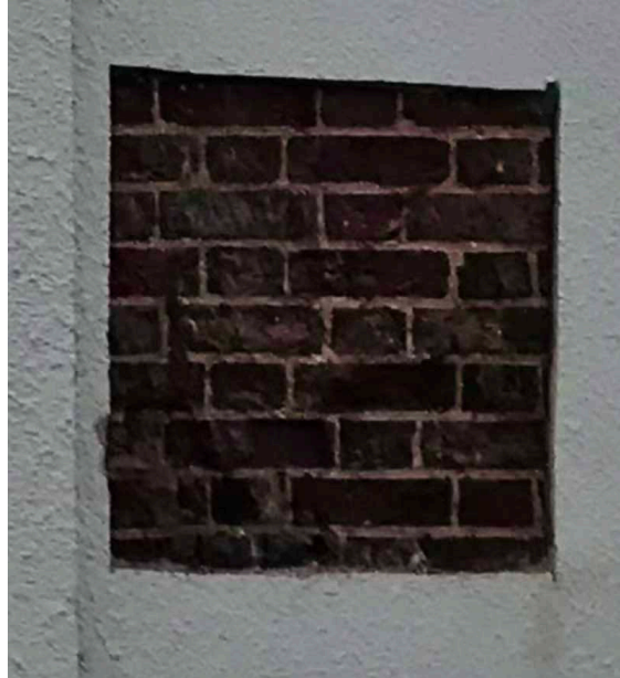
Removed patch of render reveals an attractive red brick
