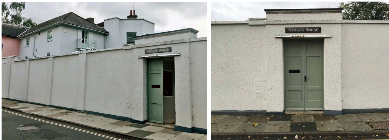
Stokes House Entrance, Ham Street
