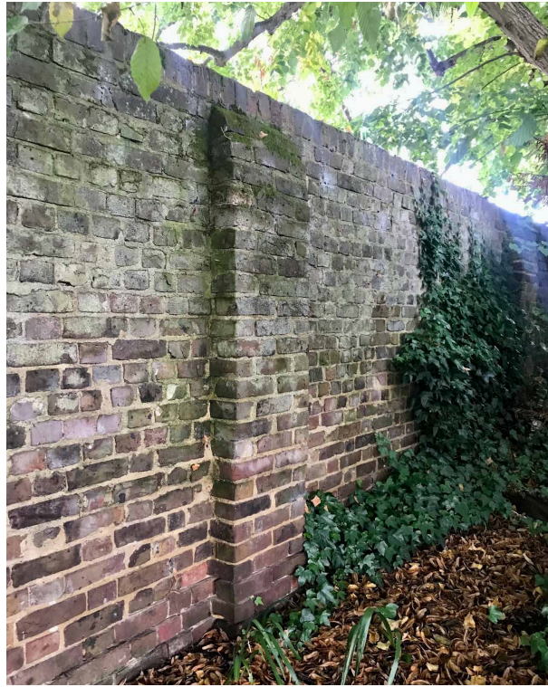
The wider piers, with less regular spacing with curved tops are thought to be earlier. Note the brick on edge along the top of the wall.
