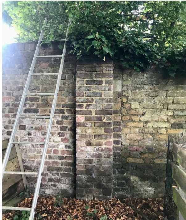
Brick wall change on northern boundary
