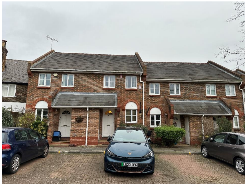
Street view of 6 Catherine Drive
