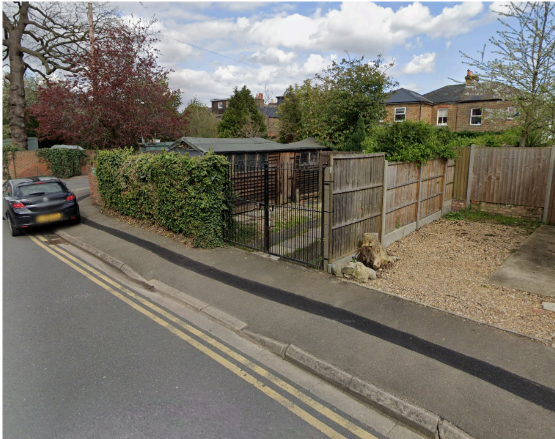
IMAGE 3: Means of Escape – Rear Garden Gate Out
