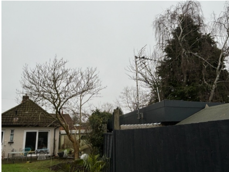
Fairlawn existing living room doors on the left with garden room roofs visible tight to boundary on right of image
