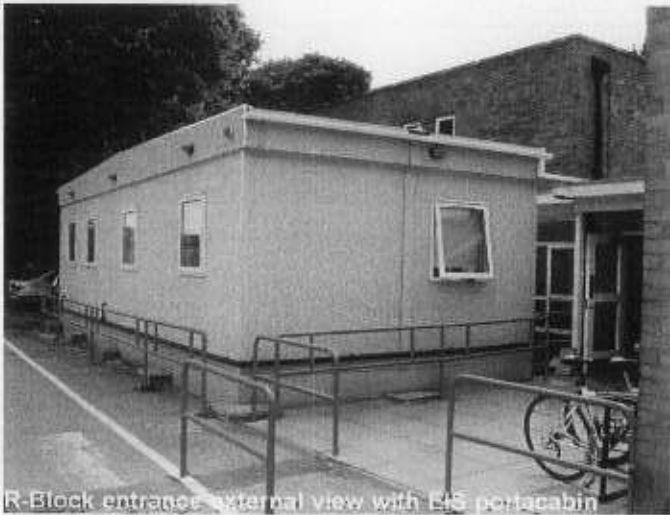
R-Block entrance external view with EIS portacabin
