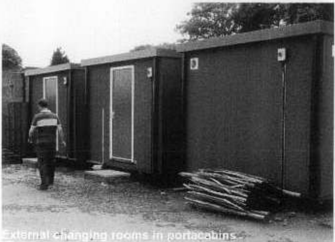
External changing rooms in portacabins
