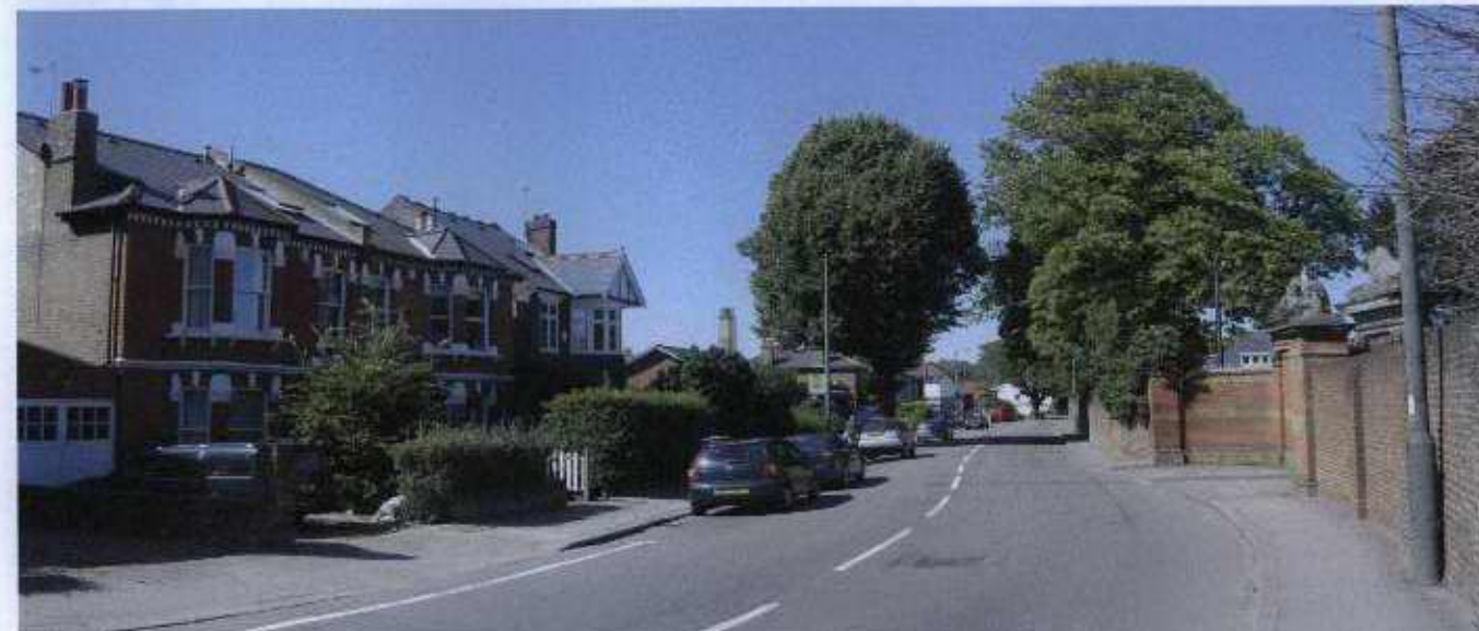
11. ST. MARGARETS ROAD FROM THE SOUTHEAST
