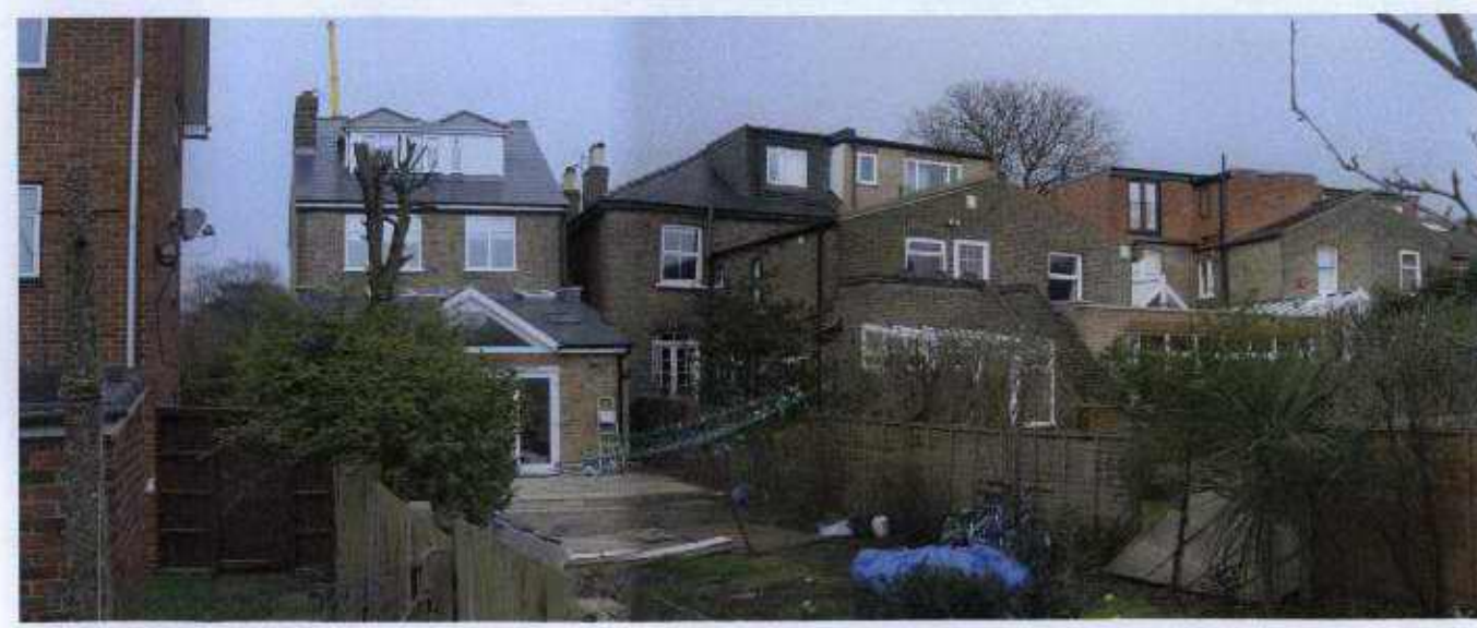
12. THE REAR OF 353-359 ST. MARGARETS ROAD, TWICKENHAM
