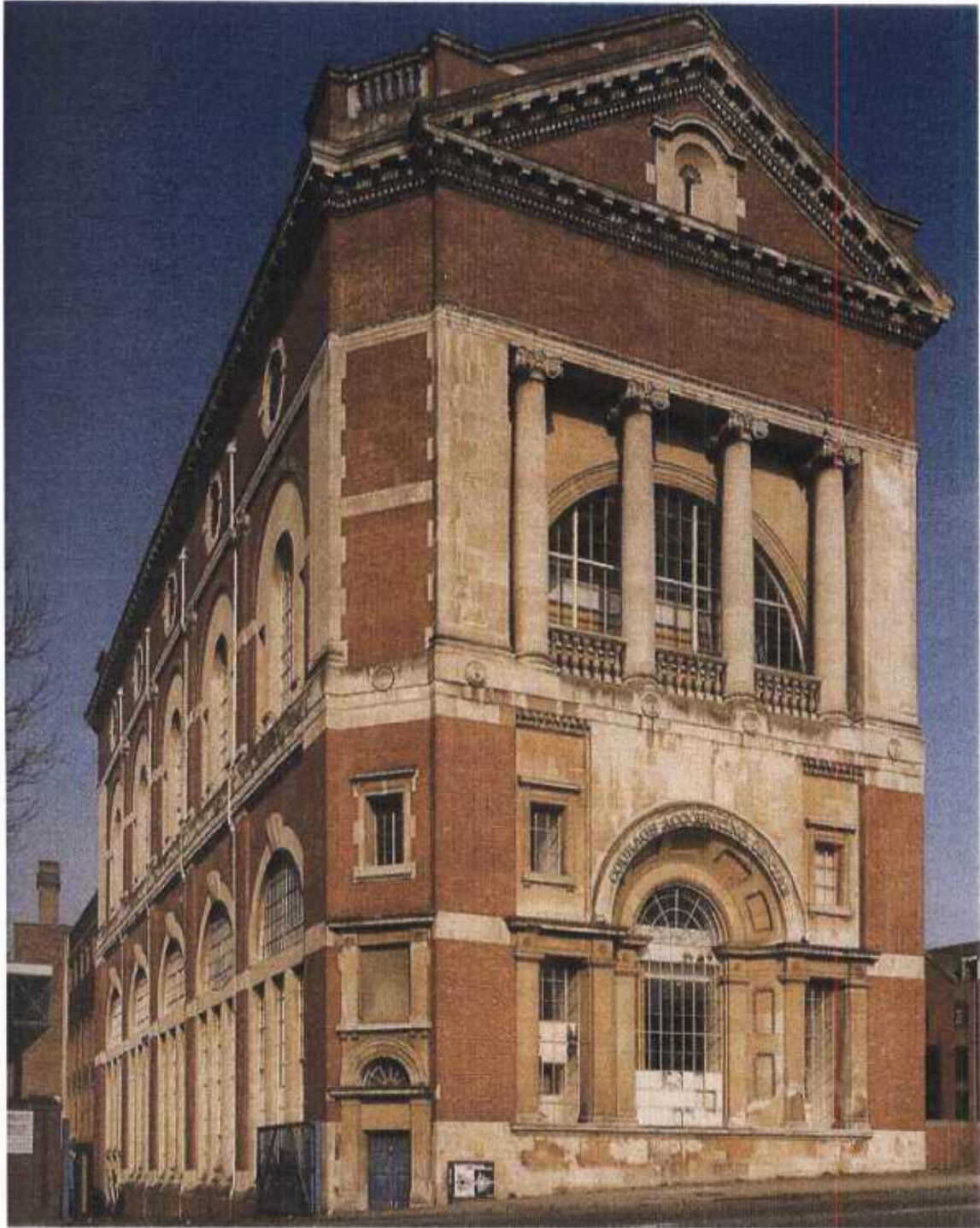
Fig. 3: Bristol Tramway and Carriage Company central generating station
