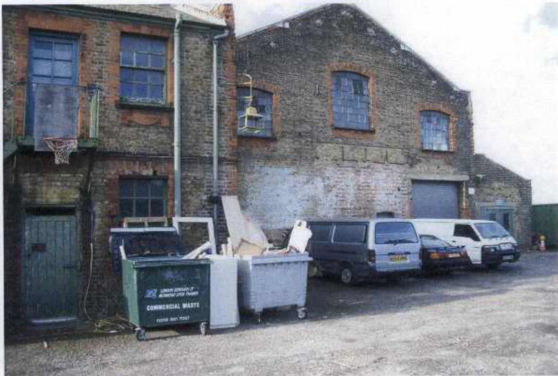
Fig. 11: The east elevation of the boiler house of the generating station at Hamilton Road, Twickenham
