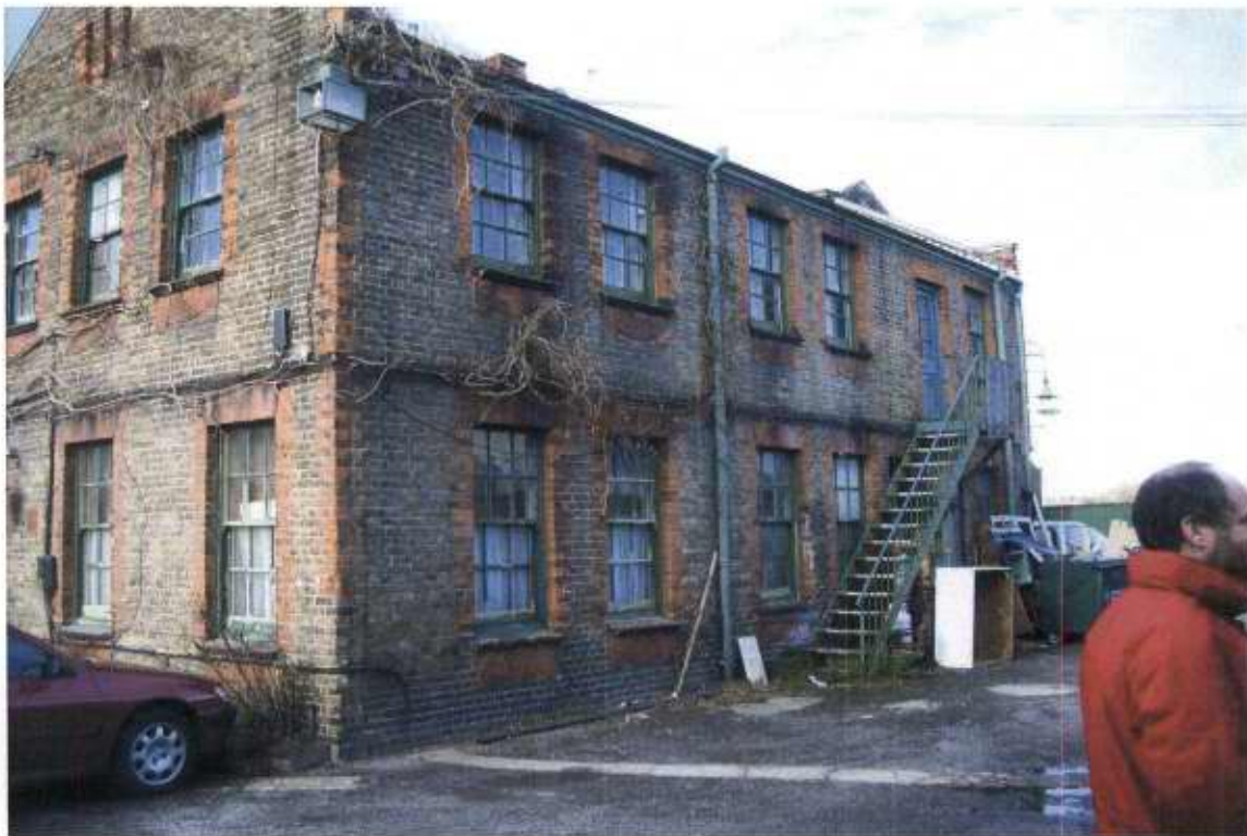
Fig. 10: The offices of the generating station at Hamilton Road, Twickenham
