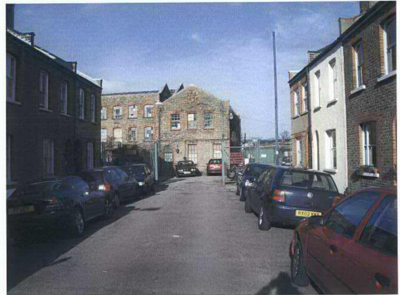
EXISTING VIEW FROM HAMILTON ROAD
