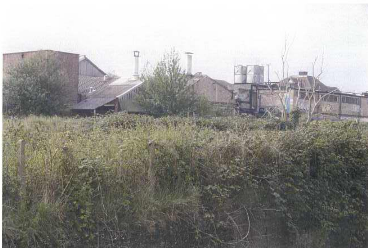
VIEW OF LARGER SCALE INDUSTRIAL BUILDINGS
