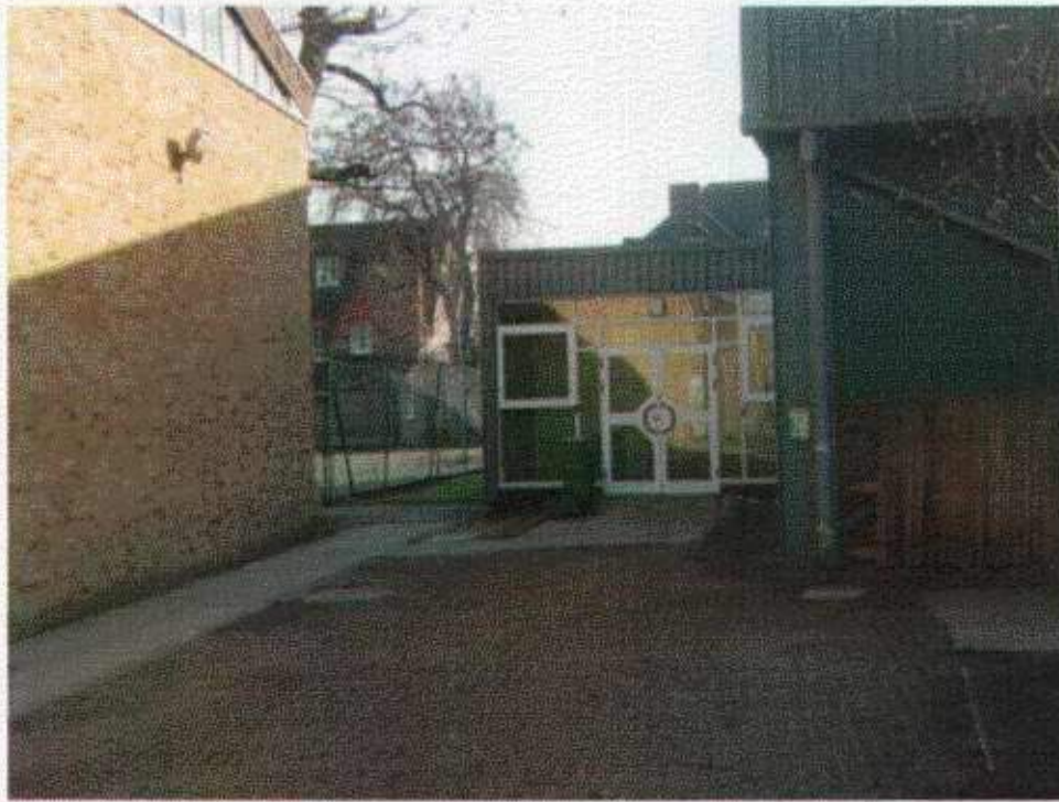
Elevation Showing Flank wall of Blocks: R (LHS) and R1 (RHS)
