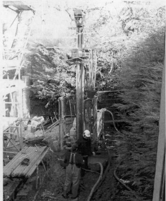
Borehole being drilled
