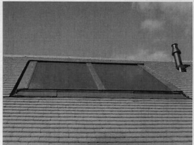
An example of a flat plate solar thermal panel
