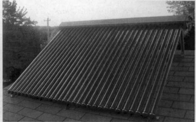
An example of an evacuated tube solar thermal module
