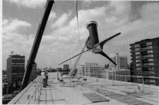
A building mounted 6kW proven wind turbine being installed
