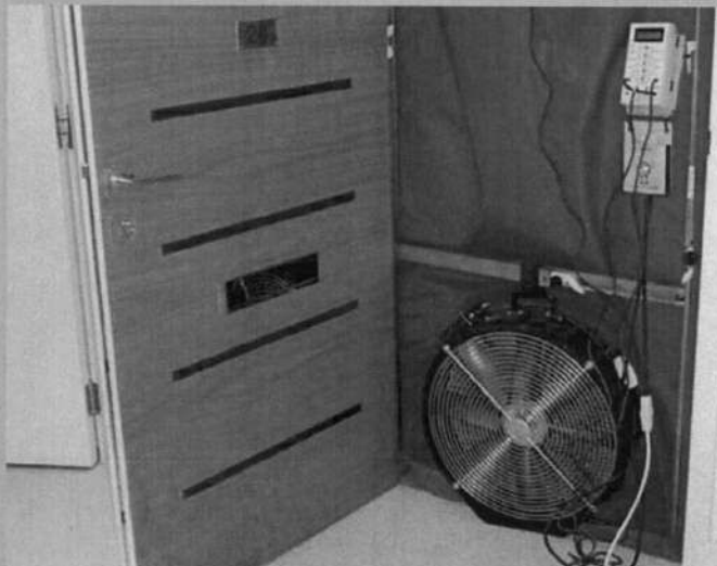
Air Tightness Test being carried out
