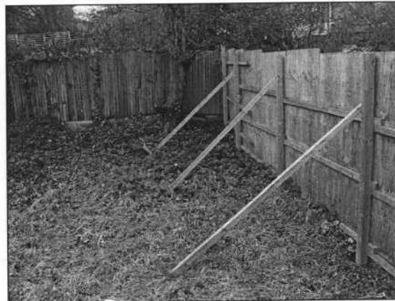
Example 2. Hoarding-style fencing with robust wooden posts with supports to ensure minimal movement.
