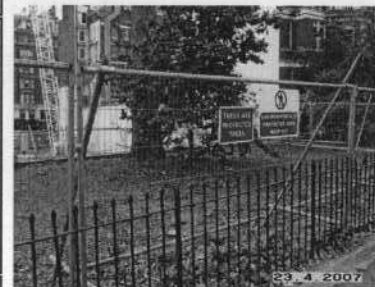
Fencing with signs
