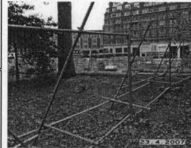
Effective fencing in position
