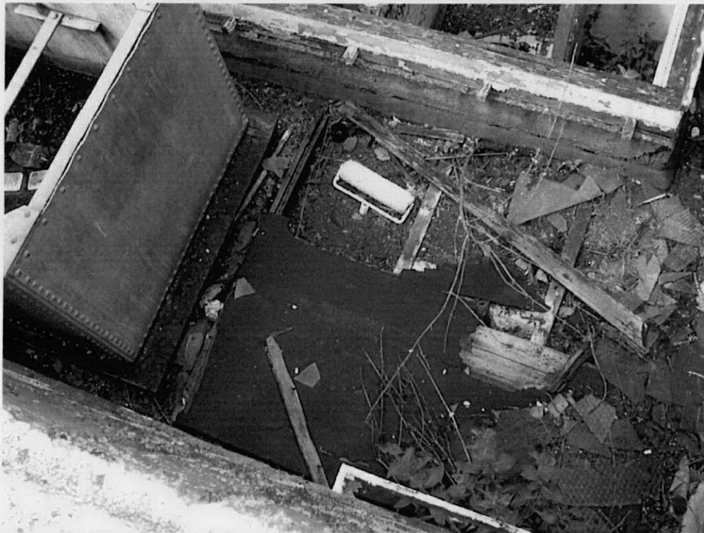
Plate 12 - Bituminous felt to roof of ladies WC (East Toilets)
