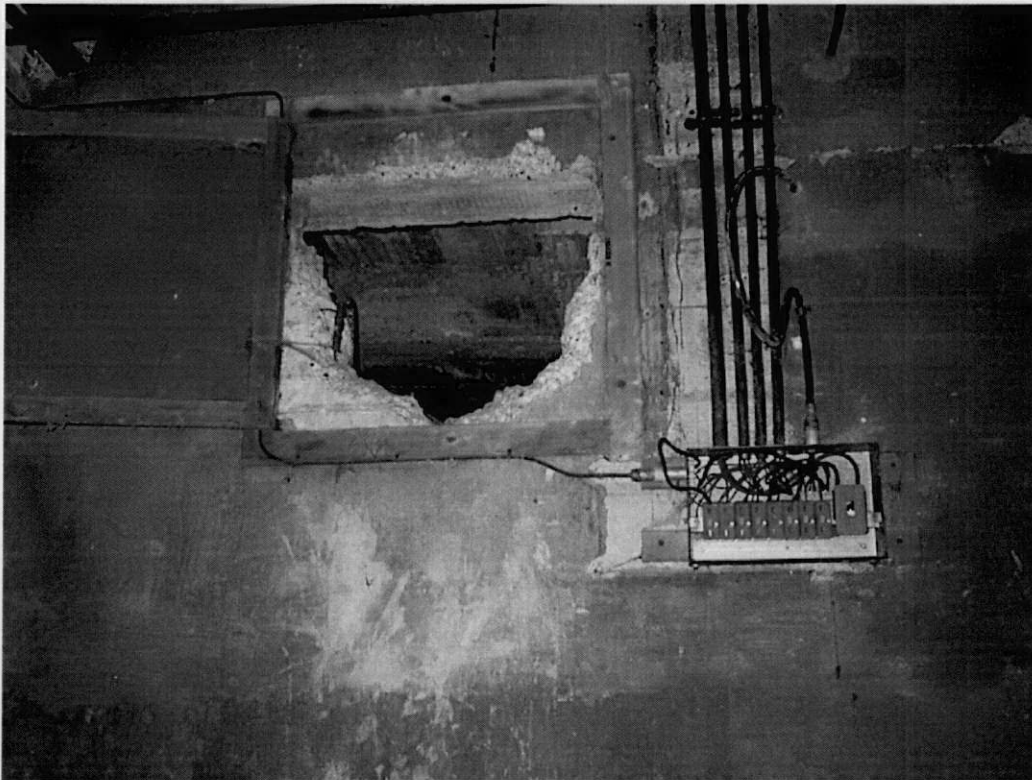
Plate 17 - Changing Block - high level access door to sub-floor void adjacent swimming pool
