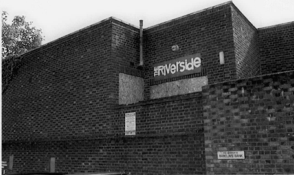
Plate 19 - Restaurant - Cement flue to northeast corner
