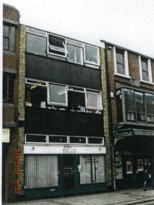
22 The Causeway. The building sits uneasily with its neighbours
