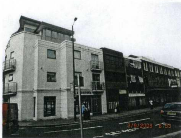
View from The Causeway with no.s 26-28 in the foreground (white rendered frontage)
