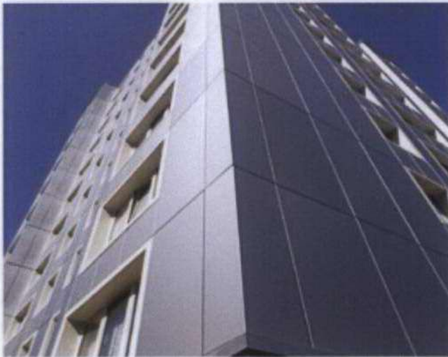
SELF COLOURED CLADDING PANELS . (by 'Trespa' or similar, colour to be approved.)
