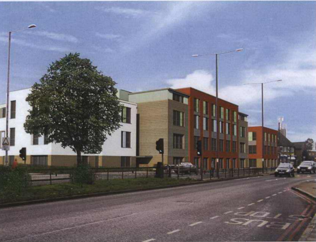
View of the junction between Lower Richmond Road and Manor Grove looking west
