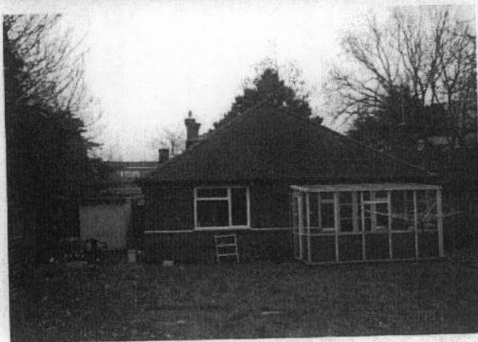
Rear elevation of 84a
