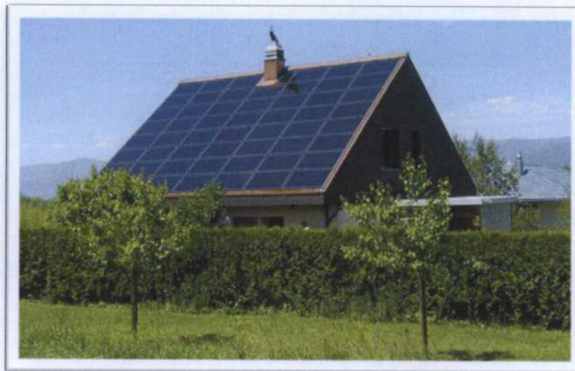
Figure 3 – A large PV array on a sloping roof
