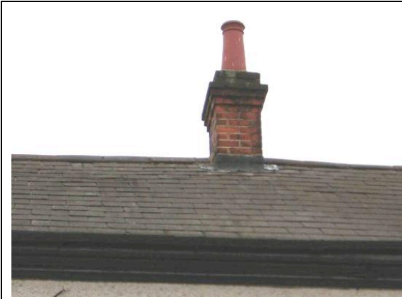
Fig. 17: Detail of eaves and chimneystack to front section
