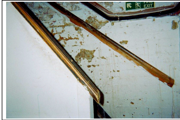
Fig. 43: Handrails from base of stairs
