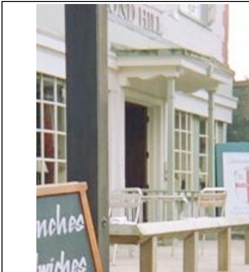
Fig. 33: Porch to main door opening
