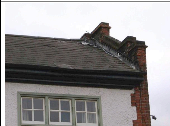
Fig. 19: View of western brick gable
