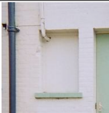
Fig. 31: Blocked window opening, east elevation
