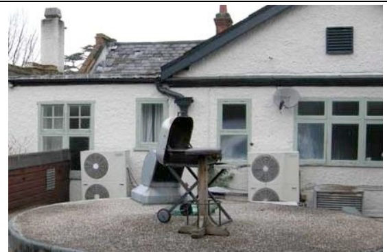
Fig. 32: Window openings, south elevation
