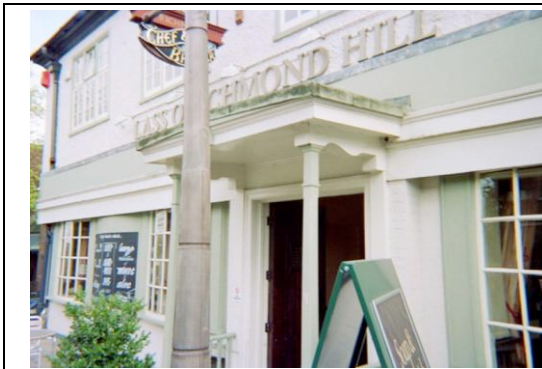
Fig. 23: Fascia and cornice added to front elevation
