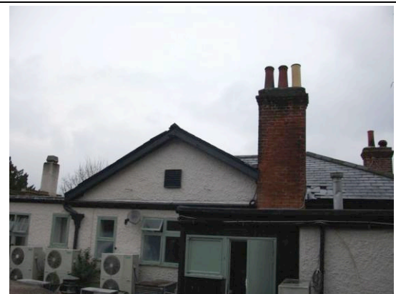
Fig. 22: Roof to rear from southeast
