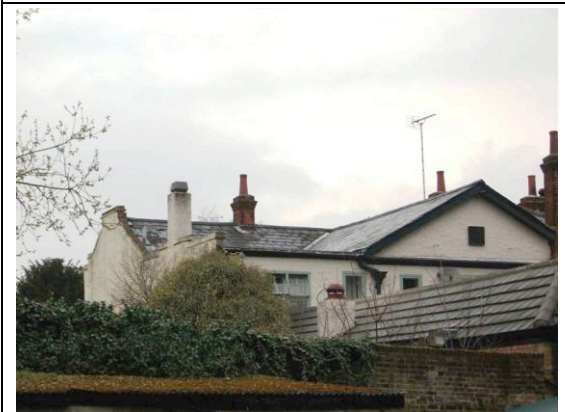
Fig. 21: Roof to rear from southwest
