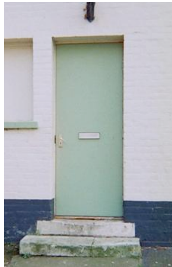
Fig. 34: Door opening, east elevation
