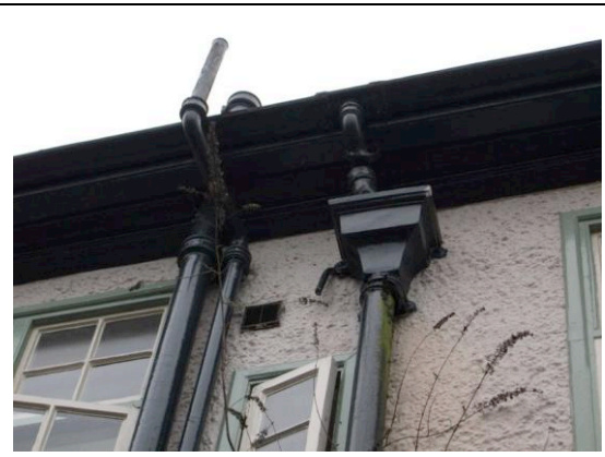
Fig. 20: Detail of rainwater goods
