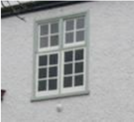
Fig. 27: First floor window opening
