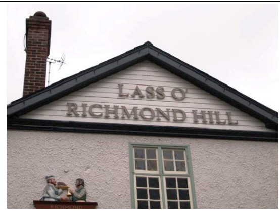
Fig. 18: View of eastern gable showing bargeboards and timber panelling
