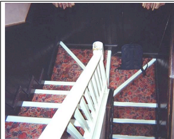
Fig. 35: Staircase from first floor landing
