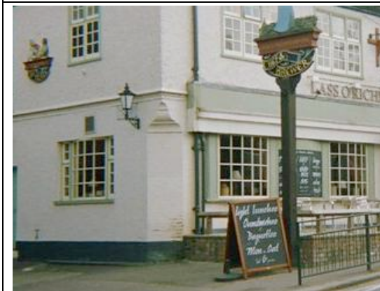
Fig. 25: Chamfer to northeast corner
