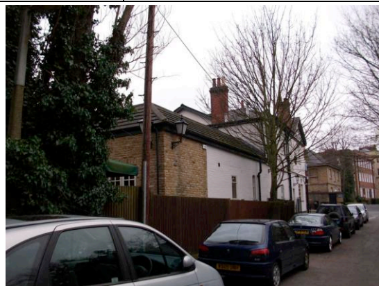
Fig. 15: east elevation from southeast
