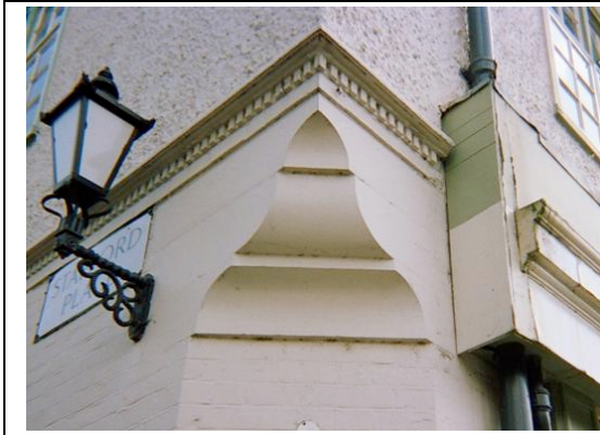
Fig. 49: Northeast corner showing truncation of stringcourse
