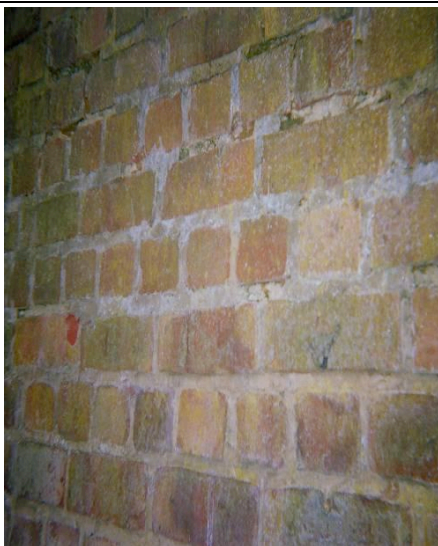
Fig. 8: A close up of the brick and failed pointing to the Park side
