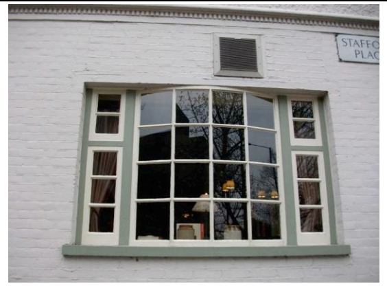
Fig. 30: Replacement window, ground floor east elevation
