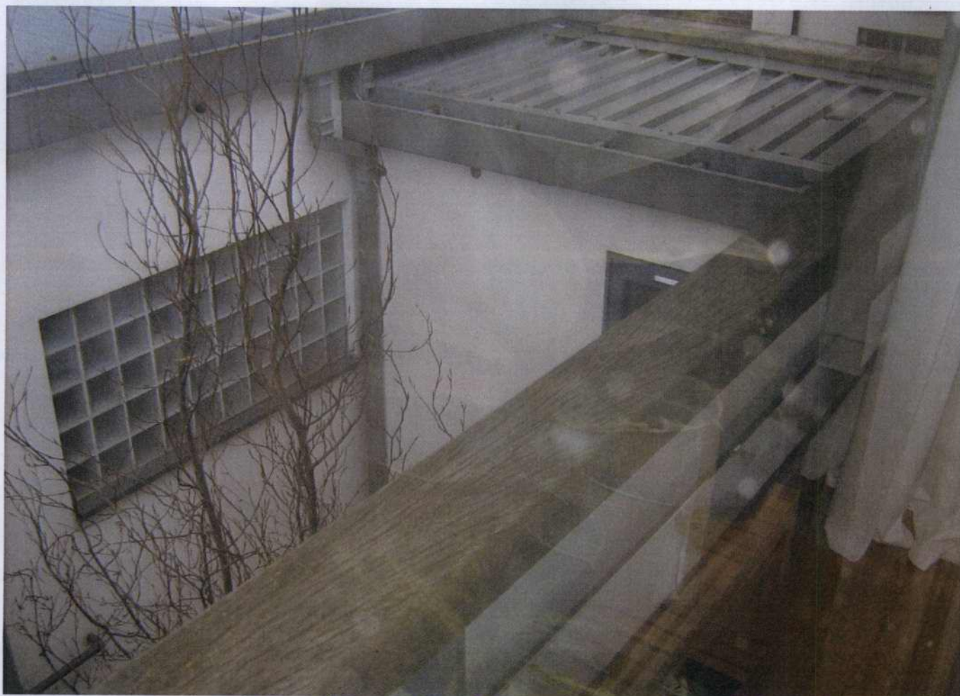
view down from lounge into MK pool courtyard
