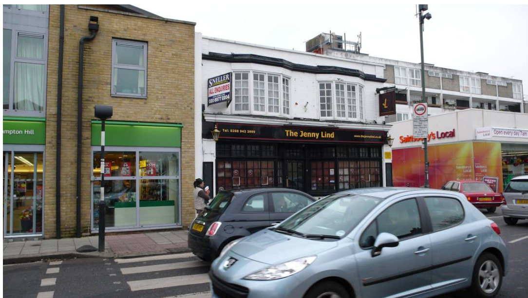
Photo 1) General view of front of site
